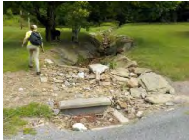
1557: The State Route 949 bridge over Callen Run is not an AOP barrier. While it does provide a slight constriction of natural streamflow, natural and semi-natural dry passage is present through both sides of the structure, as well as a semi-natural stream substrate in the channel.
