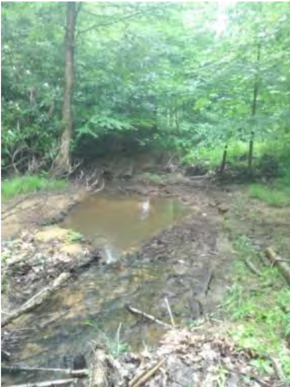
431: A relic dam (partially breached) with an old road grade on the breastworks forms a partial AOP barrier. A large sediment slug exists upstream of the breast in the former impoundment.
