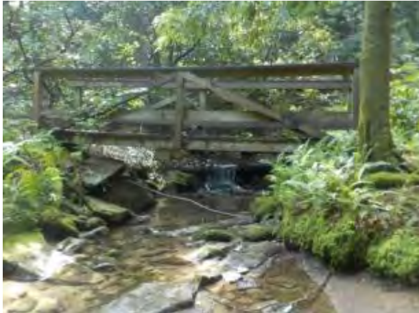
445: Several footbridges for the hiking trail in the Little Clear Creek watershed cross the stream, forming little if any AOP barrier, but still create a minor restriction on natural stream flow (left). The vehicle bridge for Corbett Road (right) is a more substantial barrier to passage for terrestrial and riparian animals, as no floodplains (dry passage) are present within the crossing structure. Crossings like these may increase animal/motorist collisions.
