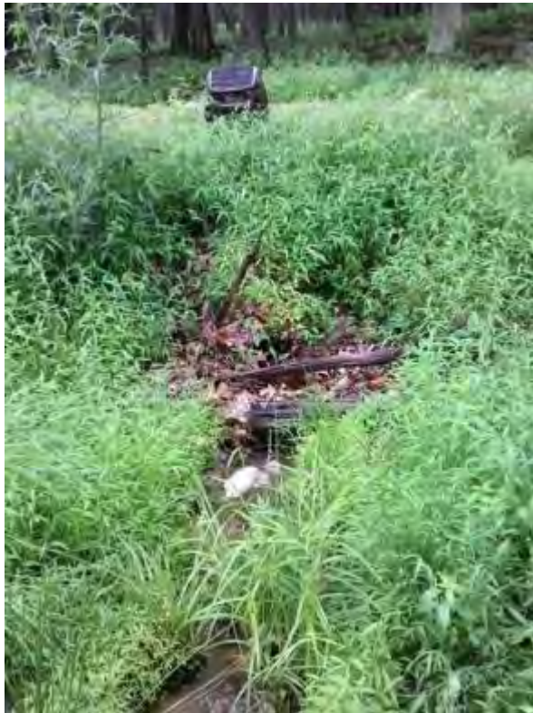
479: This crossing on a logging road in the headwaters is undersized, and therefore an AOP barrier. It is also clogged at the inlet (left). Road ditches enter directly into the stream in this area, further reducing the efficacy of the crossing structure, as well as its passability during flood flows. If the road is to continue to see use, the culvert should be replaced and DGR improvements made to reduce sedimentation to the creek.
