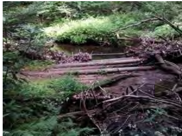
1567: A breached splash dam (left) downstream of the “upper dam” on Callen Run provides a low water AOP barrier. It is a low priority to remove, as it will likely fail on its own. A set of well casings (right) used as a foot and atv bridge has fallen into the stream, and serves as a low-water AOP barrier.
