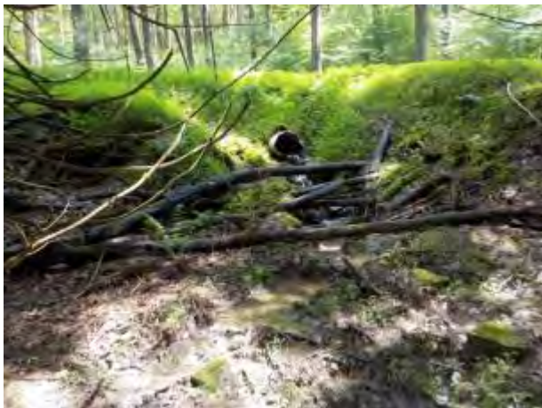
476: Two undersized culverts form AOP barriers on this stream. One is on Corbett Road (left), and the other is on Little Clear Creek Road (right). Both are perched at the outlet. Copious Japanese stiltgrass is in evidence in both of these photos.
