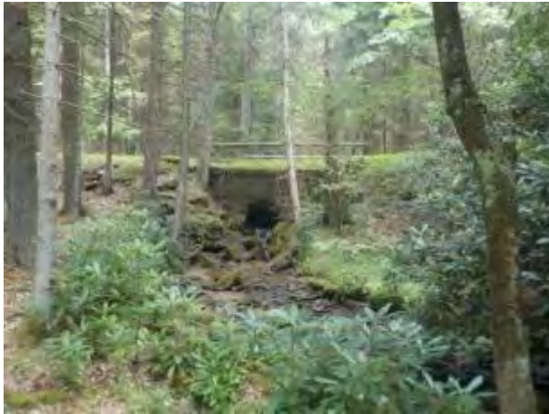
438: This undersized culvert where Clear Creek State Park Road crosses Phyllis Run prevents Aquatic organism passage from Clear Creek. The outlet is perched (left), with a large sediment slug upstream of inlet (right).
