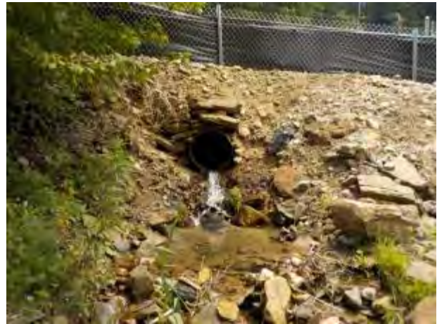
1559: Two culverts reduce connectivity on this segment. The most permanent is that which crosses under State Route 949. Its inlet (top photos) is undersized and clogged. Its outlet (middle photos) exhibits the scour pool typical of undersized crossings. Just downstream of that scour pool is the inlet to a temporary culvert (bottom left) which provides access for trucks and equipment decommissioning the Heath Pump Station. It will be removed, and this area re-contoured, at the completion of that removal and restoration project. Its outlet is perched (bottom right).
