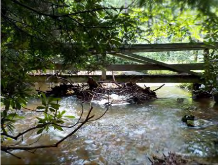
532: Smaller, mobile pieces of wood accumulating on the upstream side of this footbridge. A “catcher structure” may be a valuable upstream installation.
