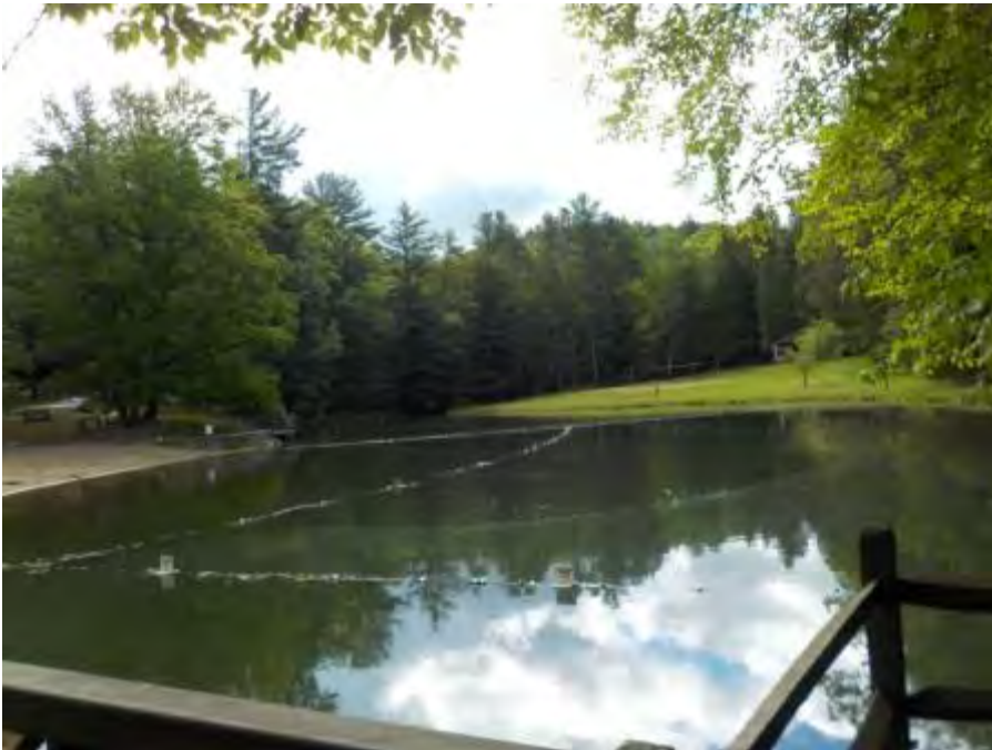
1586: One of the most noticeable AOP barriers on Clear Creek main stem is the “Swimming Dam” (above). Its high breast is a complete passage barrier to fish.
