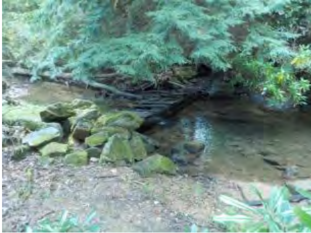
477: Two water jacks form partial to full AOP barriers at varying flow levels. The older jack (left) is falling apart. A side channel is developing to the river right of the newer jack (right), and, if properly constructed and secured, may provide passage around the jack during all flow levels.
