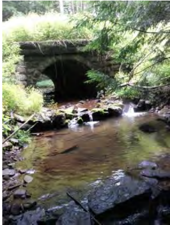
1551: Leeper Run crossing through State Route 949. Inlet (left) and outlet (right) with scour pool.
