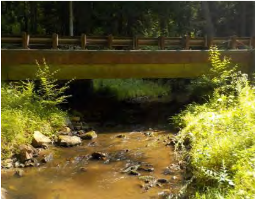
348: The Callen Run Road bridge crossing Callen Run is not a barrier to Aquatic Organism Passage. It is noted here only because it does cause a slight constriction of the floodplain, thus influencing natural stream flows in a small way.
