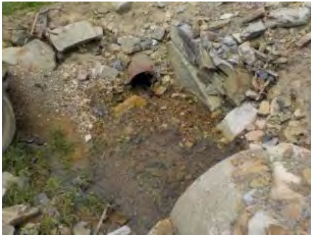
1559: Two culverts reduce connectivity on this segment. The most permanent is that which crosses under State Route 949. Its inlet (top photos) is undersized and clogged. Its outlet (middle photos) exhibits the scour pool typical of undersized crossings. Just downstream of that scour pool is the inlet to a temporary culvert (bottom left) which provides access for trucks and equipment decommissioning the Heath Pump Station. It will be removed, and this area re-contoured, at the completion of that removal and restoration project. Its outlet is perched (bottom right).
