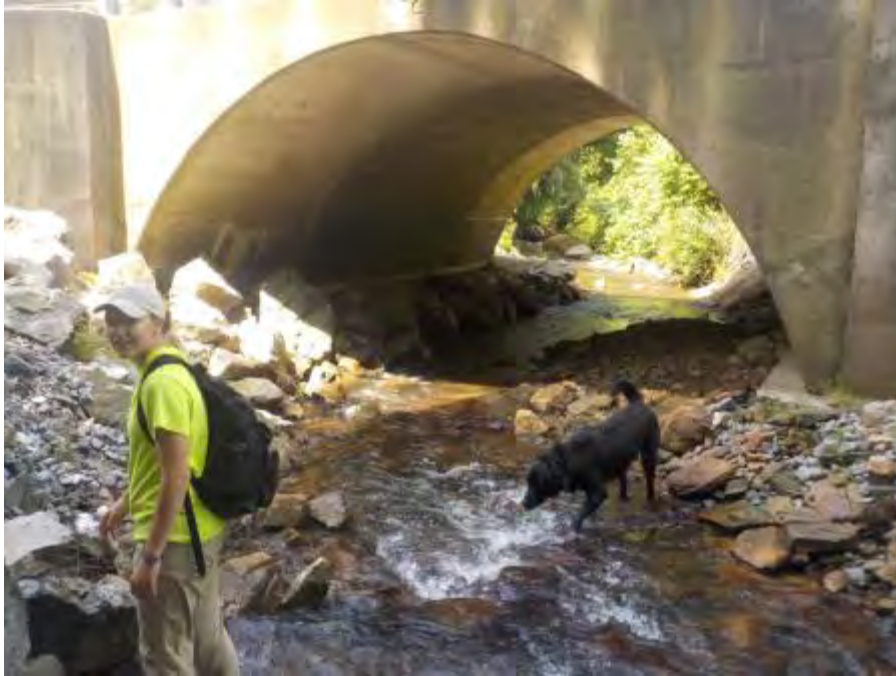
1557: The State Route 949 bridge over Callen Run is not an AOP barrier. While it does provide a slight constriction of natural streamflow, natural and semi-natural dry passage is present through both sides of the structure, as well as a semi-natural stream substrate in the channel.
