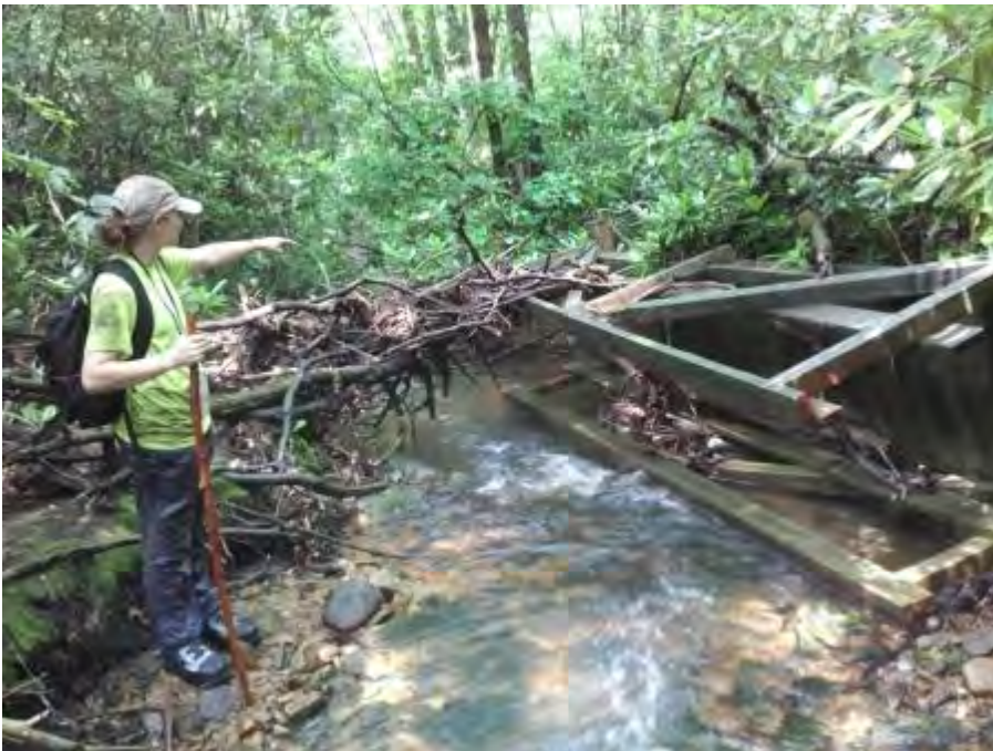
532: Smaller, mobile pieces of wood accumulating on the upstream side of this footbridge. A “catcher structure” may be a valuable upstream installation.
