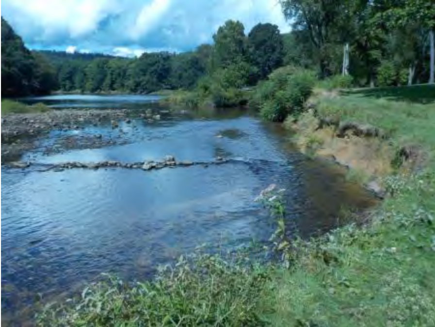
Clarion River at the confluence with Clear Creek: Though not technically one of the streams assessed in the Coldwater Conservation Plan, the Clarion River immediately downstream of the mouth of Clear Creek has been experiencing significant erosion for several years. Note the constructed riffle or “hand dam” directing flow toward the eroding bank, which is a part of Clear Creek State Park.
