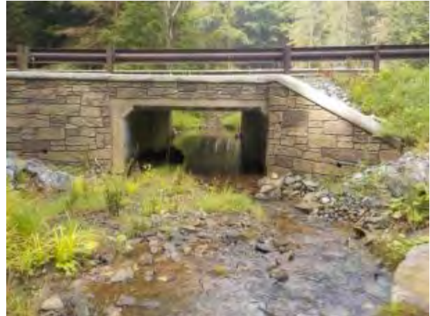
445: Several footbridges for the hiking trail in the Little Clear Creek watershed cross the stream, forming little if any AOP barrier, but still create a minor restriction on natural stream flow (left). The vehicle bridge for Corbett Road (right) is a more substantial barrier to passage for terrestrial and riparian animals, as no floodplains (dry passage) are present within the crossing structure. Crossings like these may increase animal/motorist collisions.
