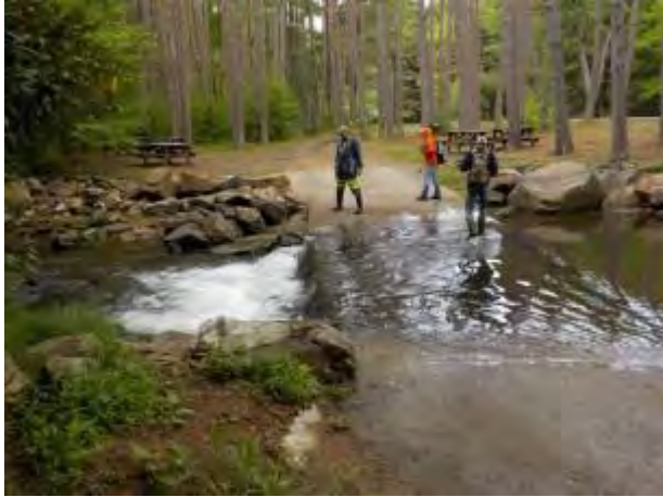
439: Two barriers to fish passage on Clear Creek main stem include a vehicle ford to a picnic area and a jack dam.
