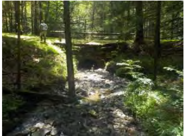
438: This undersized culvert where Clear Creek State Park Road crosses Phyllis Run prevents Aquatic organism passage from Clear Creek. The outlet is perched (left), with a large sediment slug upstream of inlet (right).
