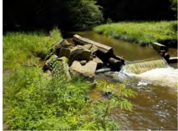
477: Two water jacks form partial to full AOP barriers at varying flow levels. The older jack (left) is falling apart. A side channel is developing to the river right of the newer jack (right), and, if properly constructed and secured, may provide passage around the jack during all flow levels.
