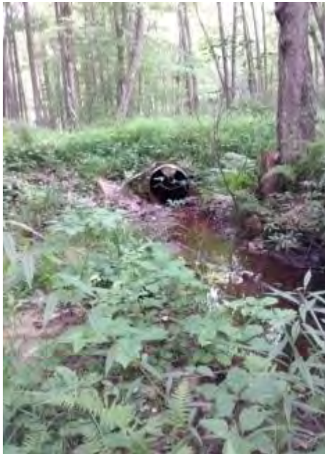
490: The culvert on Callen Run Road, where it crosses Callen Run in the headwaters, is undersized. A sediment wedge is forming upstream of the inlet (left), and the outlet is perched (right). Downstream of the outlet's primary scour area, sediment from the dirt and gravel road has begun to accumulate.
