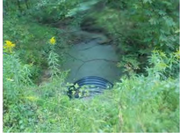
570: Shaffer Road Culvert. Inlet with sediment slug (left), Outlet with scour pool (right).
