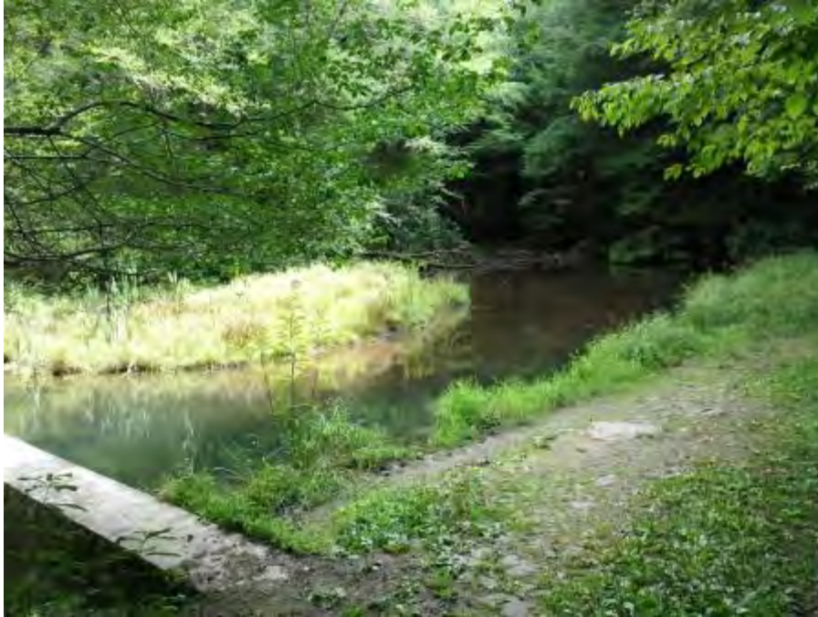
1567: Impoundment with sediment upstream of the upper dam on Callen.
