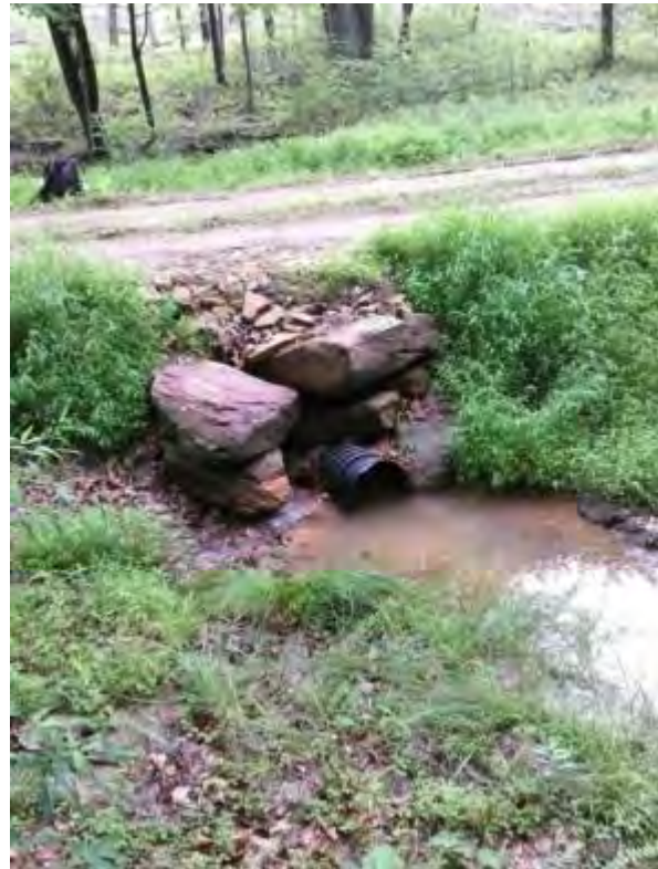
479: This crossing on a logging road in the headwaters is undersized, and therefore an AOP barrier. It is also clogged at the inlet (left). Road ditches enter directly into the stream in this area, further reducing the efficacy of the crossing structure, as well as its passability during flood flows. If the road is to continue to see use, the culvert should be replaced and DGR improvements made to reduce sedimentation to the creek.
