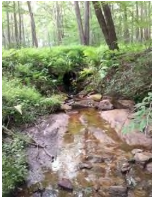
490: The culvert on Callen Run Road, where it crosses Callen Run in the headwaters, is undersized. A sediment wedge is forming upstream of the inlet (left), and the outlet is perched (right). Downstream of the outlet's primary scour area, sediment from the dirt and gravel road has begun to accumulate.
