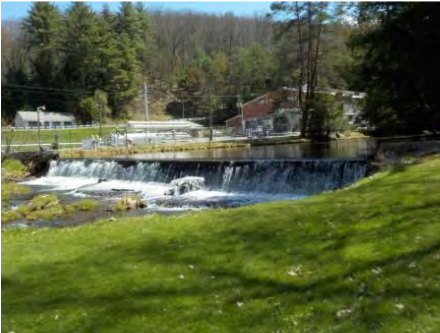
1561: Callen Run Dam during a high water event.
