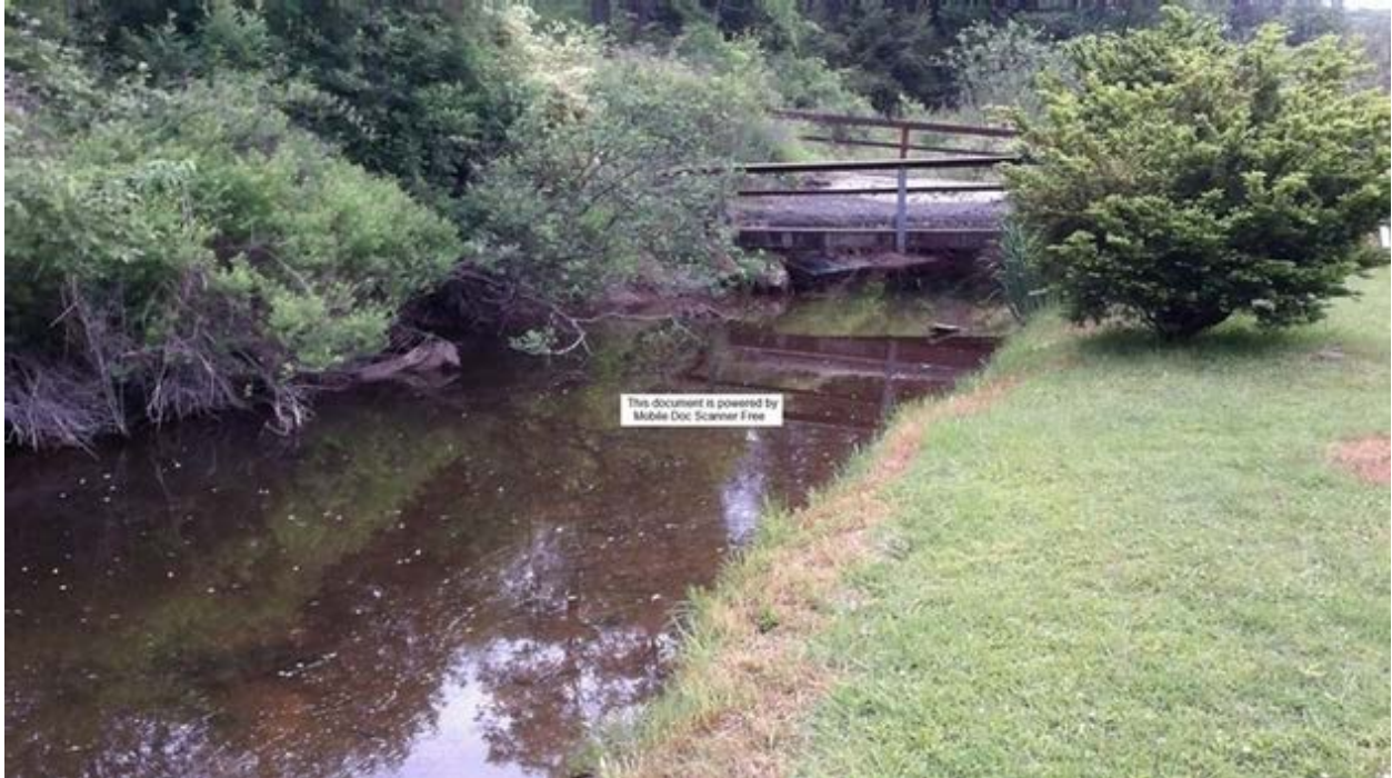
Figure 24. Road-stream crossing on Old Ellenton Mountain Road prior to flooding event.
