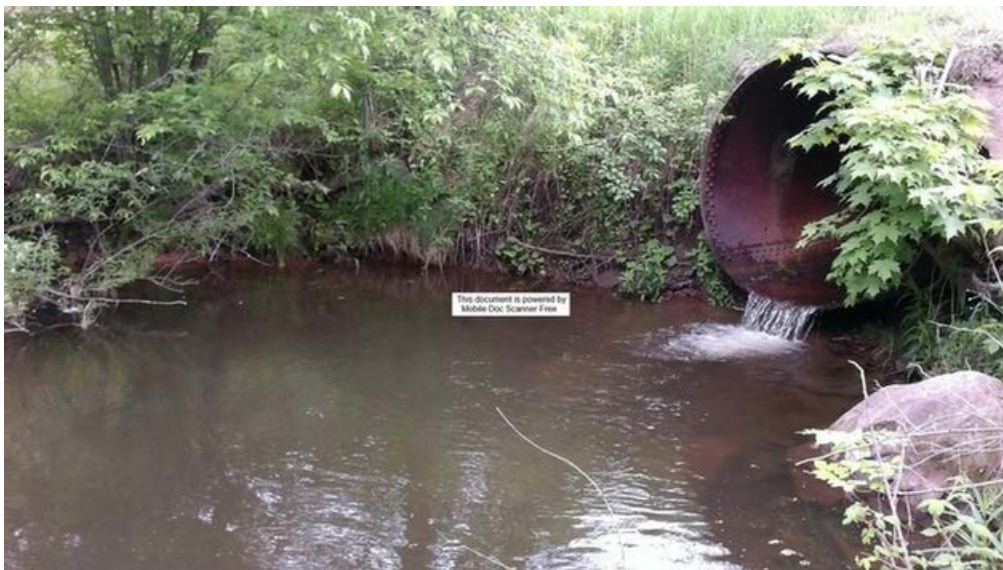
Figure 22. Culvert on Hawk Run (outlet)
