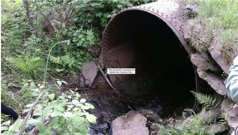
Figure 21. Culvert on Hawk Run (inlet)
