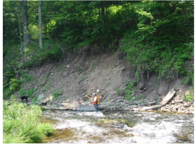
FIGURE 4. Severe bank erosion where the stream channel is along the valley slopes
