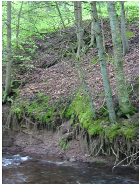
FIGURE 30. Trout Run bank erosion near road.
