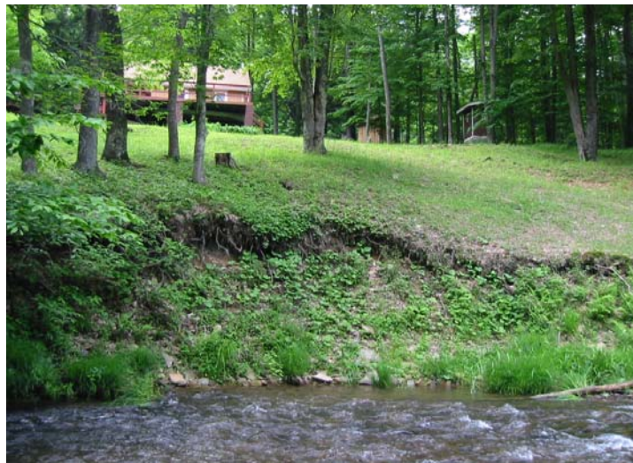
FIGURE 27. Cross Fork erosion downstream of Yochum Run.
