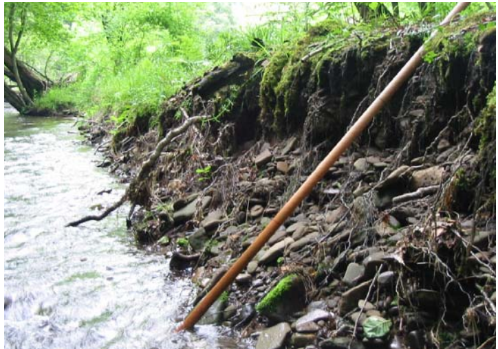
FIGURE 29. Bank erosion on Yochum Run.
