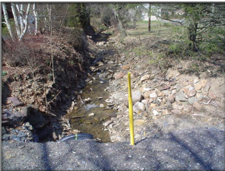
Site # 10: Looking upstream from the highway cross-drain.
