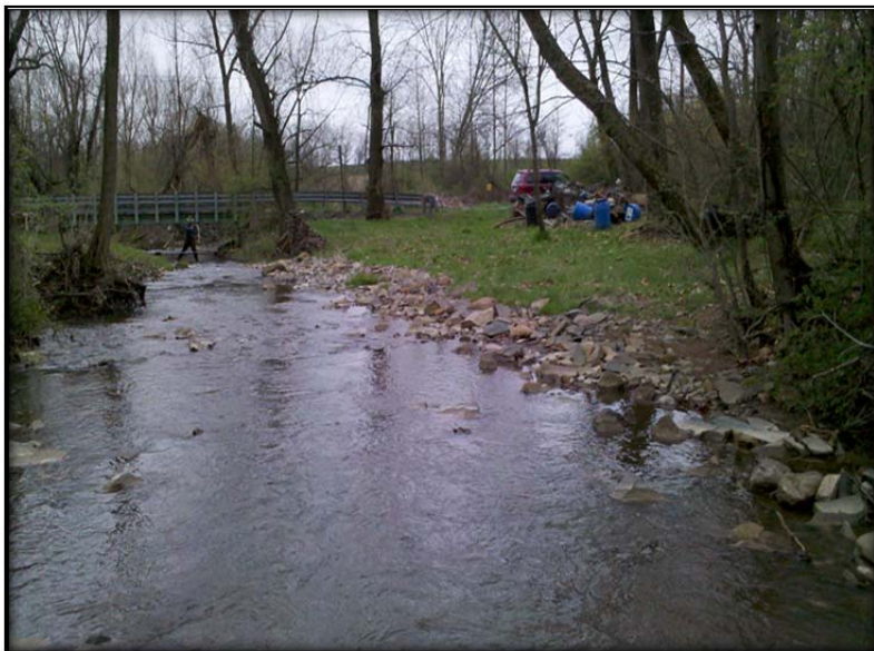
Site #1: Upstream from the bridge.
