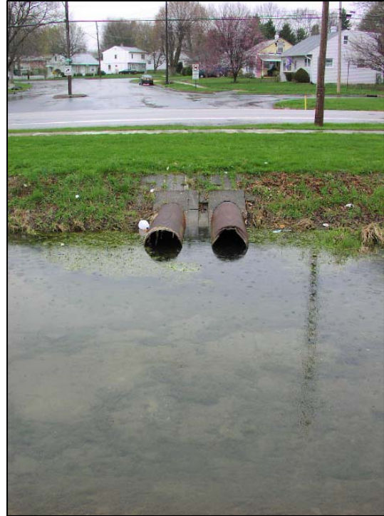
Stormwater pipes flow directly into Cedar Run across from the Allen Middle School
