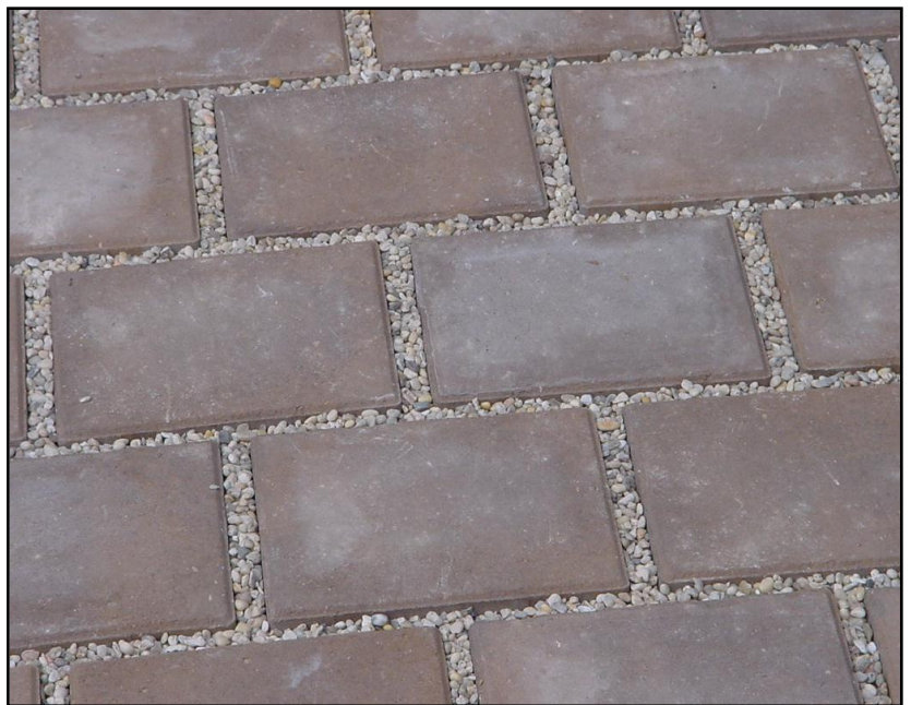
Porous pavers, like these installed at the Dauphin County Agriculture and Natural Resource Center, allow rain to infiltrate into the ground, instead of becoming runoff.
