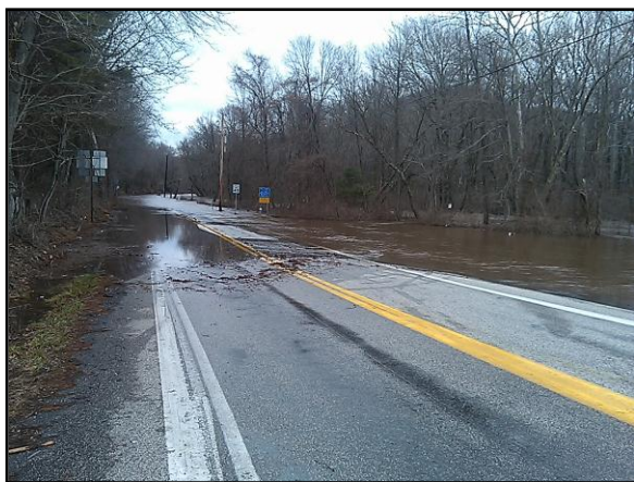
Flooding near site CLRK 0185 in early March 2011
