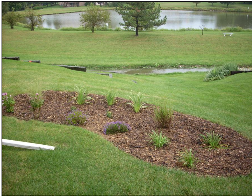
The rain garden helps to infiltrate and control stormwater
