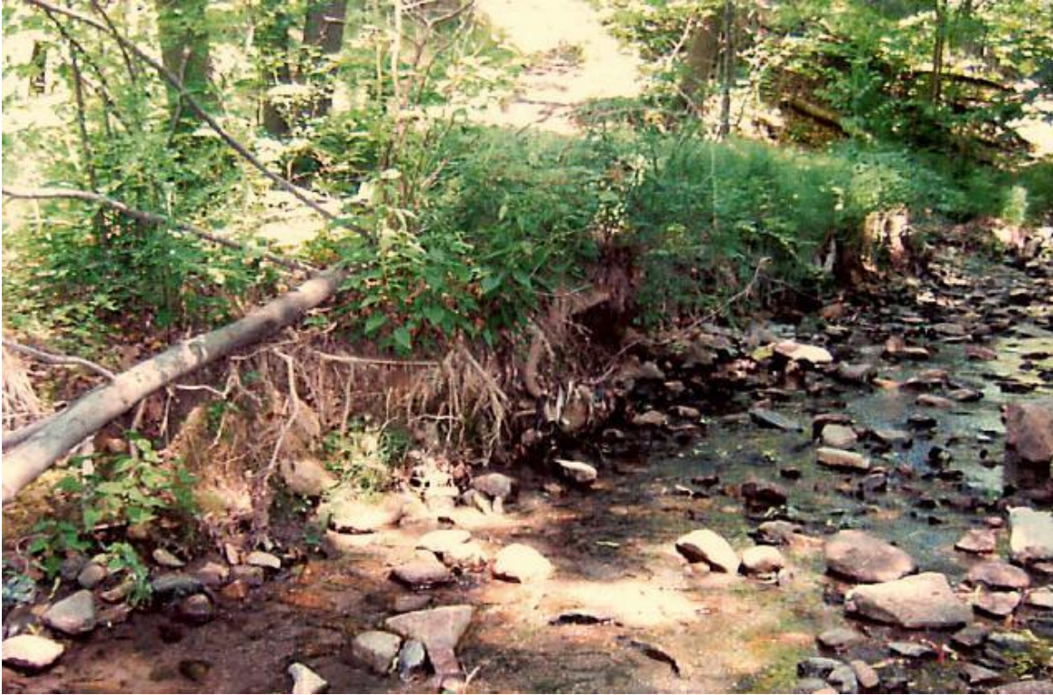
Banks show increased erosion where the creek has continued to widen.
