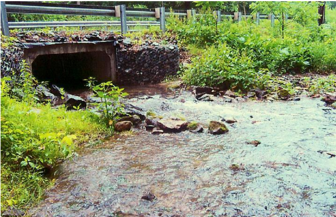
Creek is channeled to flow under the bridge culvert and then allowed to expand back to its natural course.
