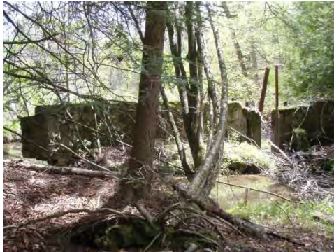
6231: Clockwise from top left: Relic, breached dam upstream of State Route 66; box culvert on State Route 66-minimal floodplain development inside; Relic, breached dam downstream of State Route 66; another view of the same breached dam downstream of SR 66. These dams are partial/minimal AOP barriers.
