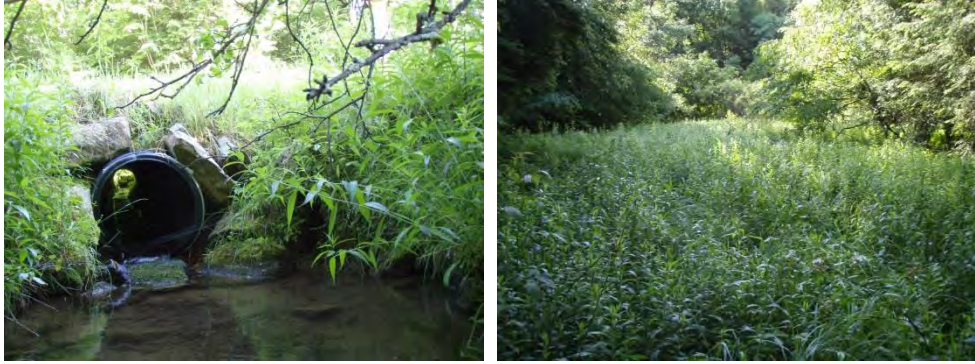
6110: Undersized culvert at West Kane Road (left); sedimented basin of relic log pond (right).
