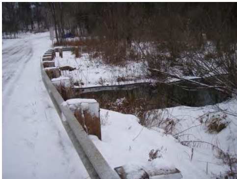
7200: Bridge at top of segment constricts flow, no floodplain development underneath.
