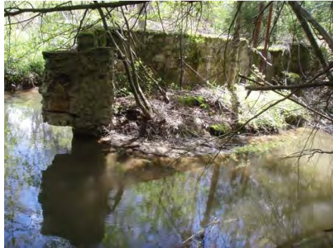
6231: Clockwise from top left: Relic, breached dam upstream of State Route 66; box culvert on State Route 66-minimal floodplain development inside; Relic, breached dam downstream of State Route 66; another view of the same breached dam downstream of SR 66. These dams are partial/minimal AOP barriers.
