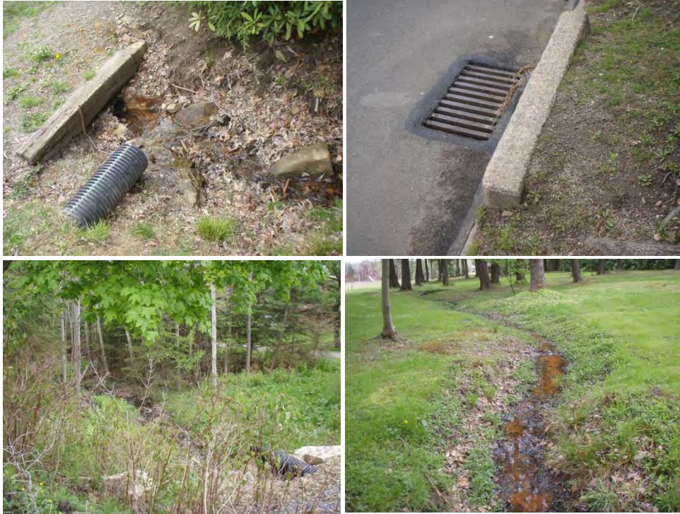
6090: Clockwise from Top Left: Stream enters urban stormwater system from headspring in Evergreen Park; street stormwater grate draining directly to stream; small discolored tributary in Evergreen Park; Stream exits culverted stormwater system, with Japanese knotweed in foreground.
