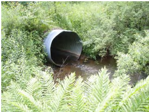
6105: Relic log dam forms partial AOP barrier (top left), Reigel Road culverts (top right), private road culvert (bottom left).
