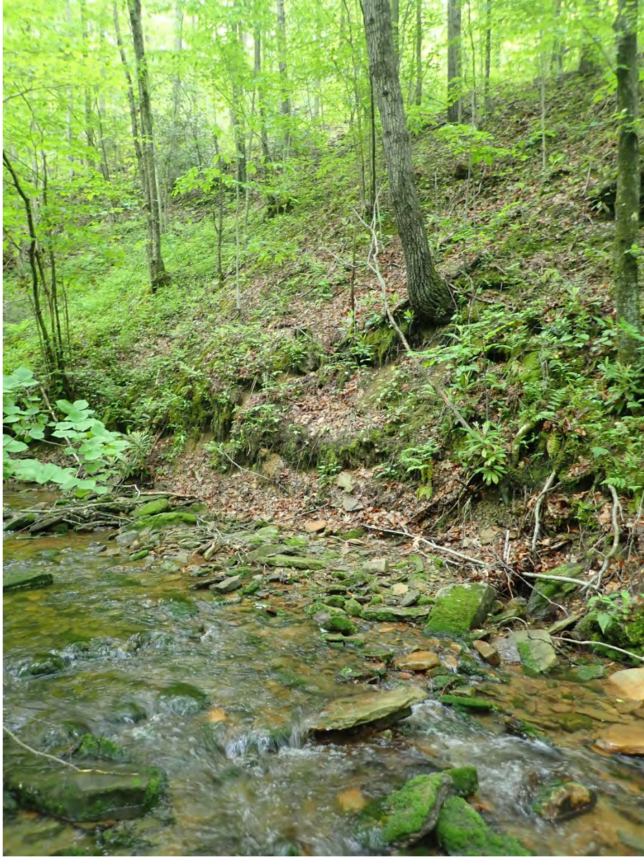
Photo 7. Mild erosion on the left bank.
