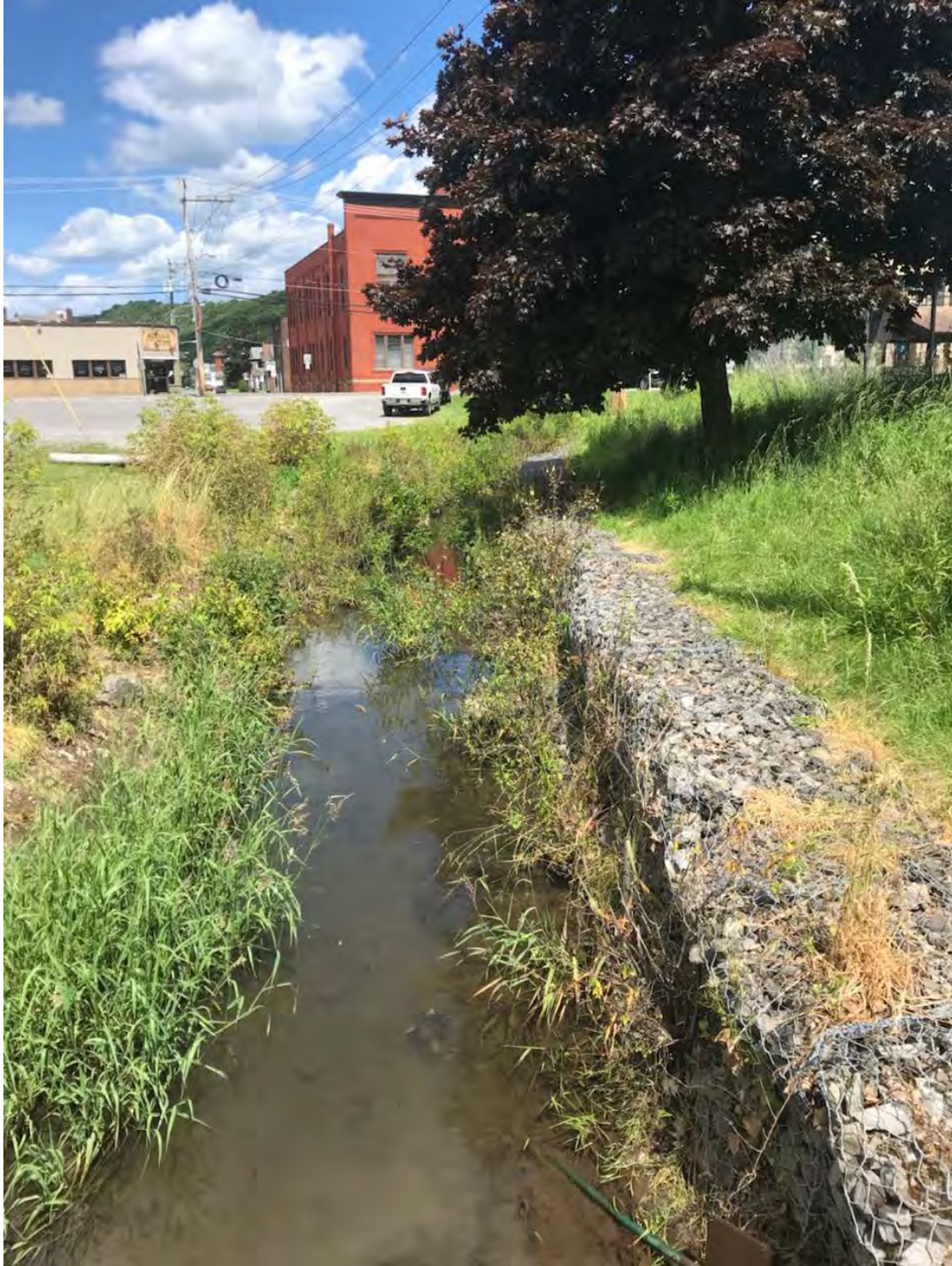
Photo 21. Looking upstream at Aiello's Café from the Ridgway YMCA basketball courts. The stream through this segment of the property is entirely lined by gabion baskets and lacks instream habitat.
