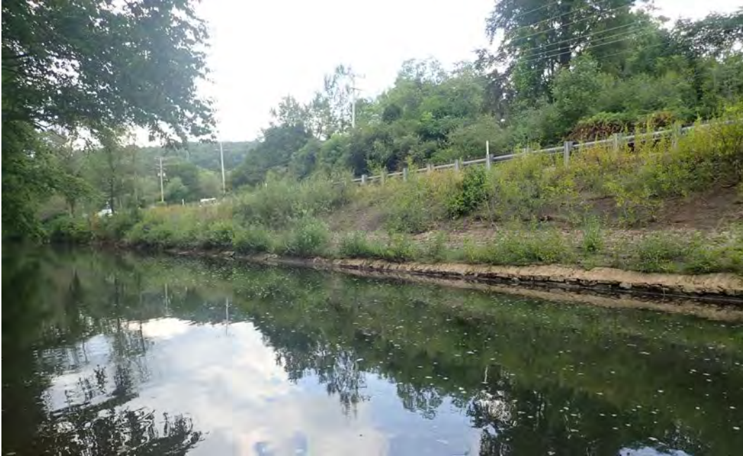
Photo 136. Cement reinforced bank along Highway 120 in EC18.
