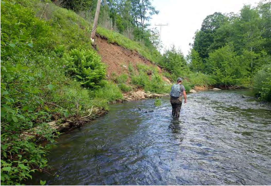
Photo 72. Left bank erosion along the powerline right-of-way in EC02.
