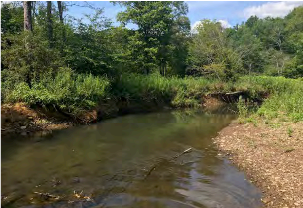
Photo 61. Left bank erosion in EC12 which could be stabilized by root wad deflectors.
