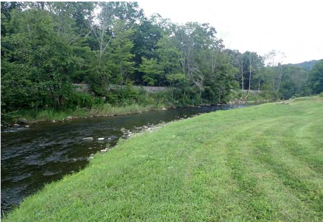
Photo 135. EC18 flowing along the railroad by Ridgway Powered Metals. The railroad elevation creates a lewy barrier and does not allow water passage.
