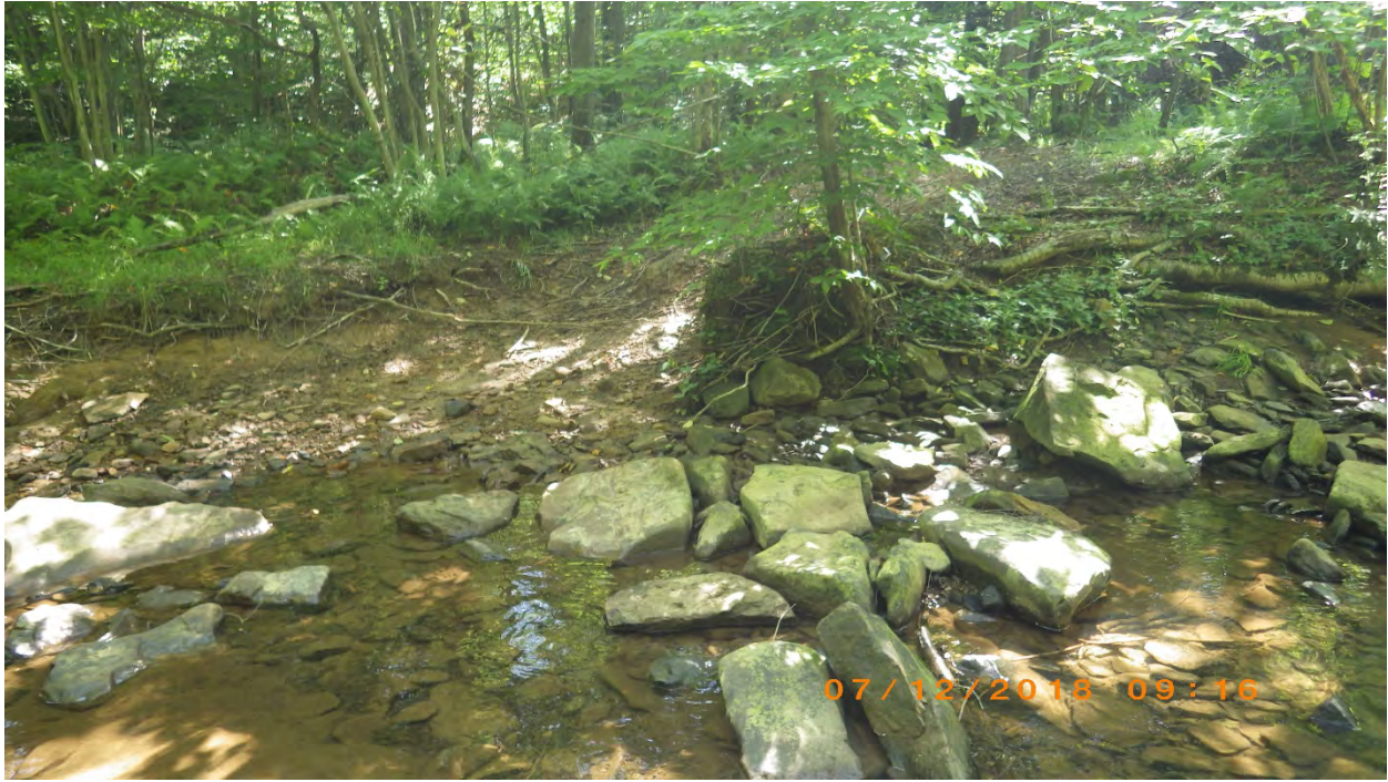
Photo 31. Right bank erosion in LR09 caused by ATV trail erosion.
