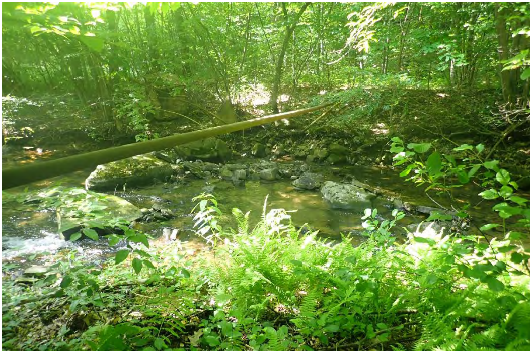
Photo 27. Pipeline crossing the stream channel in MR05.
