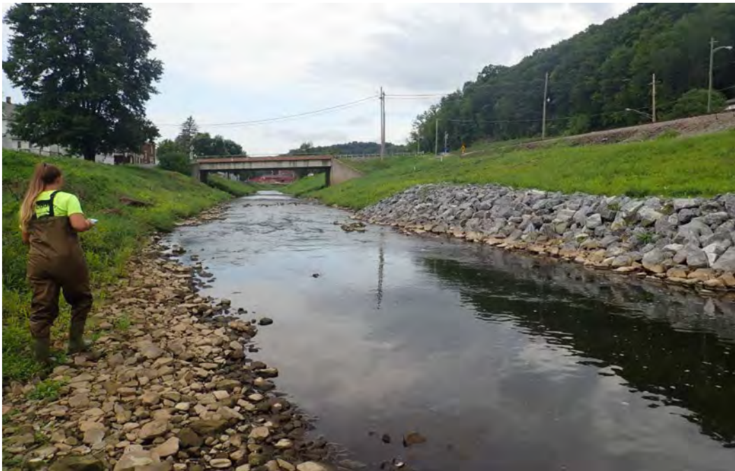
Photo 147. Riprap bank stabilization upstream from the Broad Street bridge.
