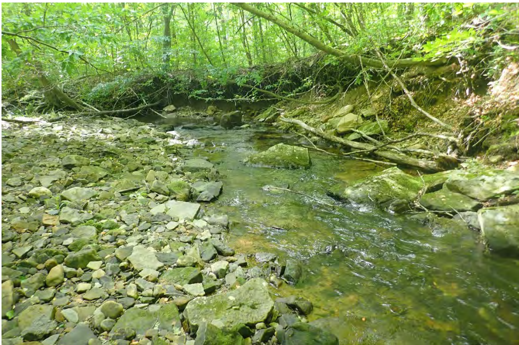
Photo 21. Eroded and undercut left bank in MR05.
