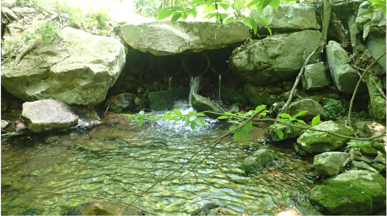
Photo 1. Outlet of culvert immediately upstream from the Daguscahonda/Decker Run confluence.
