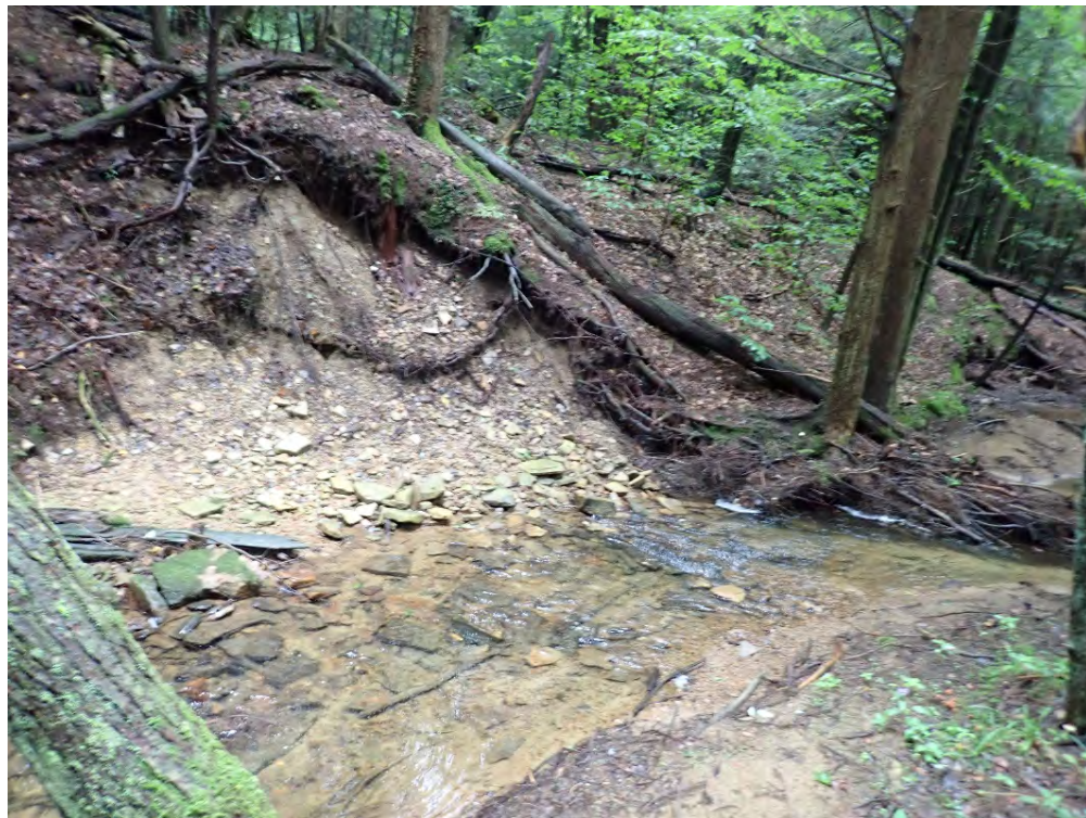
Photo 4. Approximately 12ft high eroding left bank in SR01.
