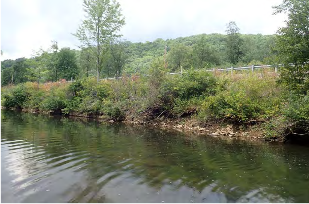
Photo 130. Highway 120 encroachment on EC18.
