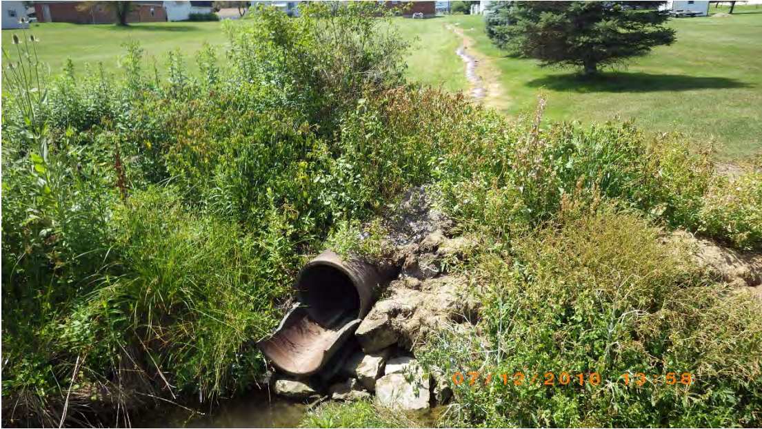
Photo 6. French drain from a private residence which outlet to UNT to IR01.
