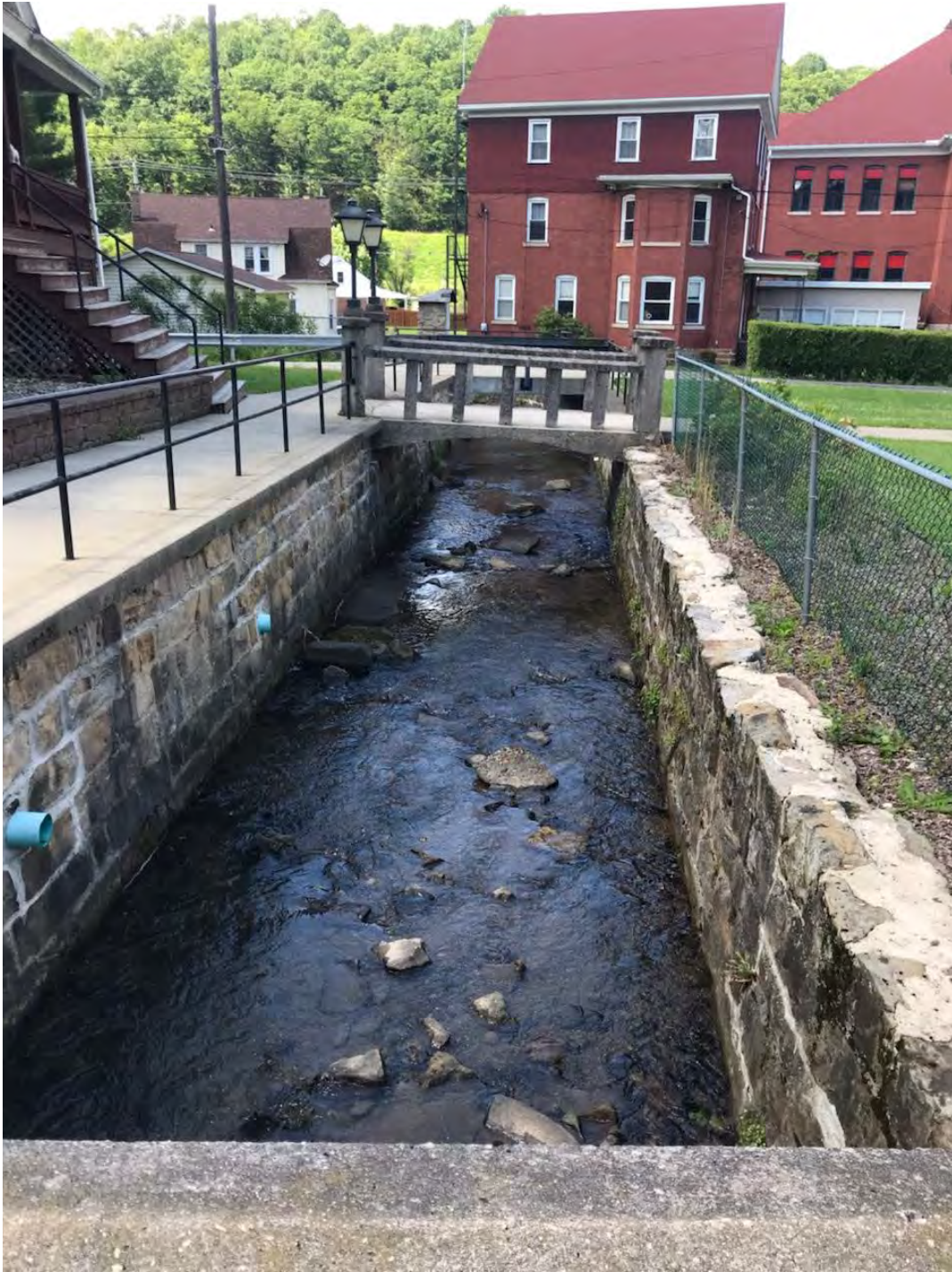
Photo 19. Looking downstream as Gallagher Run flows through St. Leo's Catholic School property. Drains that outlet immediately into the stream channel (left) do not allow for settling and assimilation of stormwater contaminates before reaching the stream.
