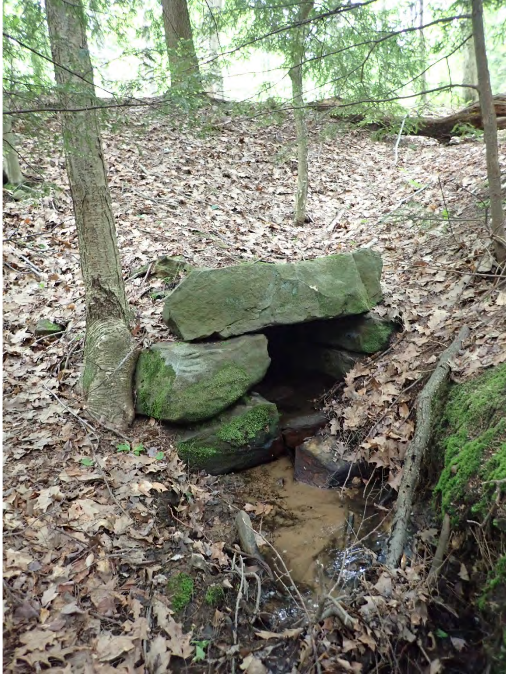
Photo 1. Beginning of Gallagher Run from spring landscaped with boulders.
