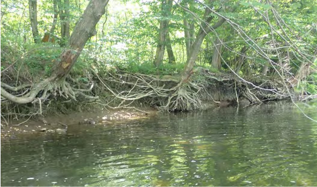
Photo 122. Eroded bank downstream of the Highway 120 bridge over EC17.
