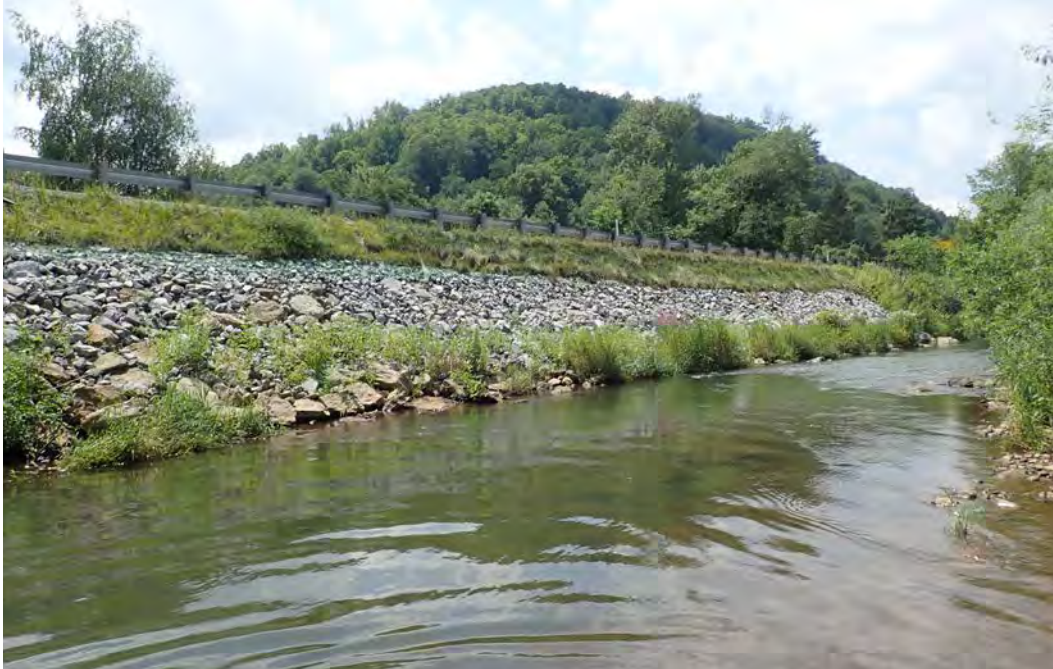
Photo 98. Riprap bank reinforcement along Highway 120 in the town of Daguscahonda.
