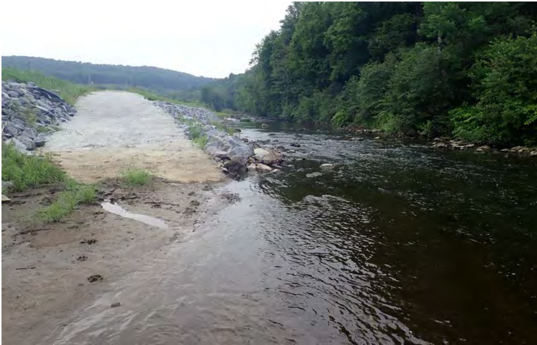
Photo 145. Creek access ramp behind the PennDOT building.
