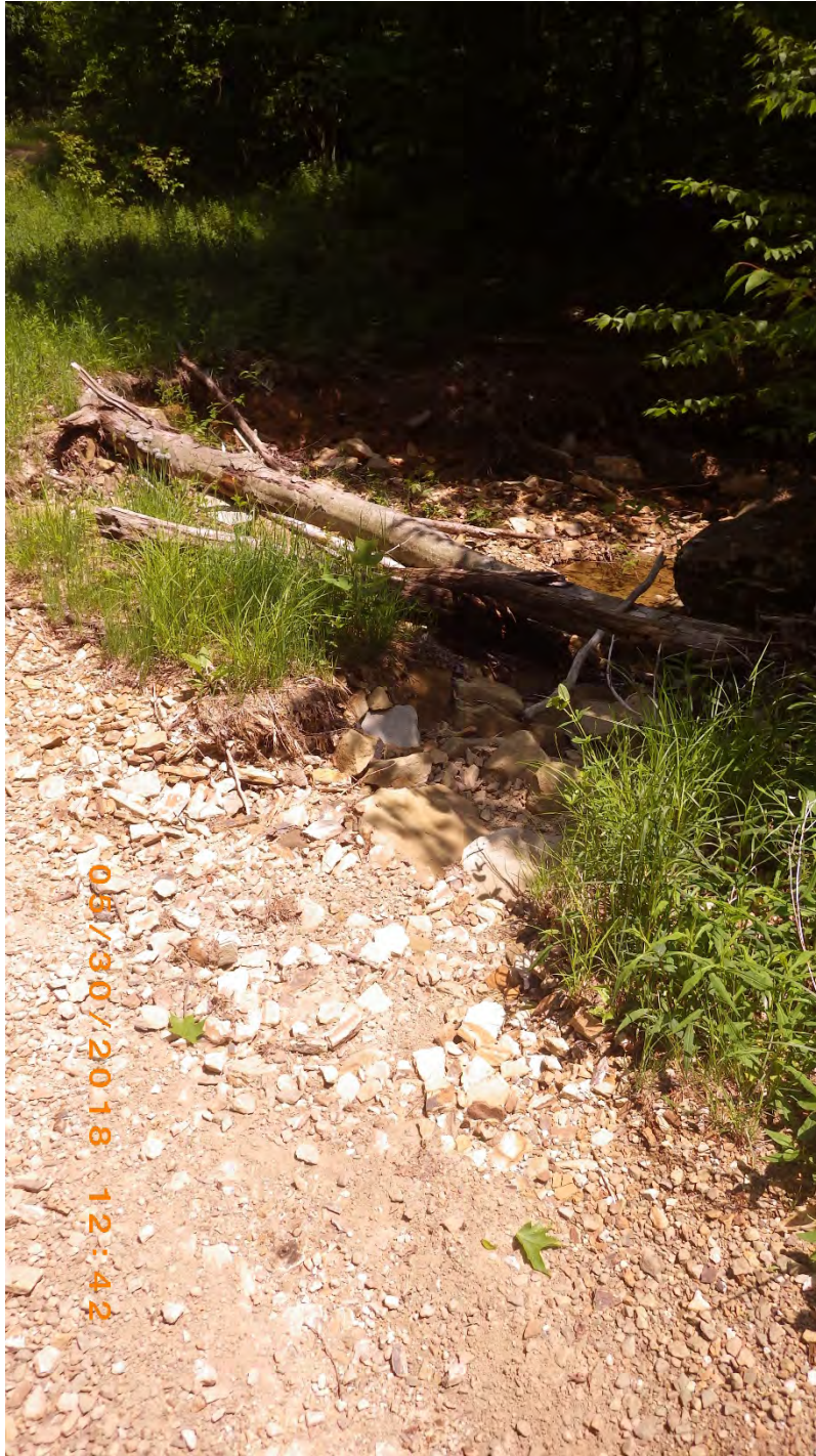
Photo 4. Erosion from gravel road. Water leaving the gravel road removed sediment from the road surface and deposited it into the stream.
