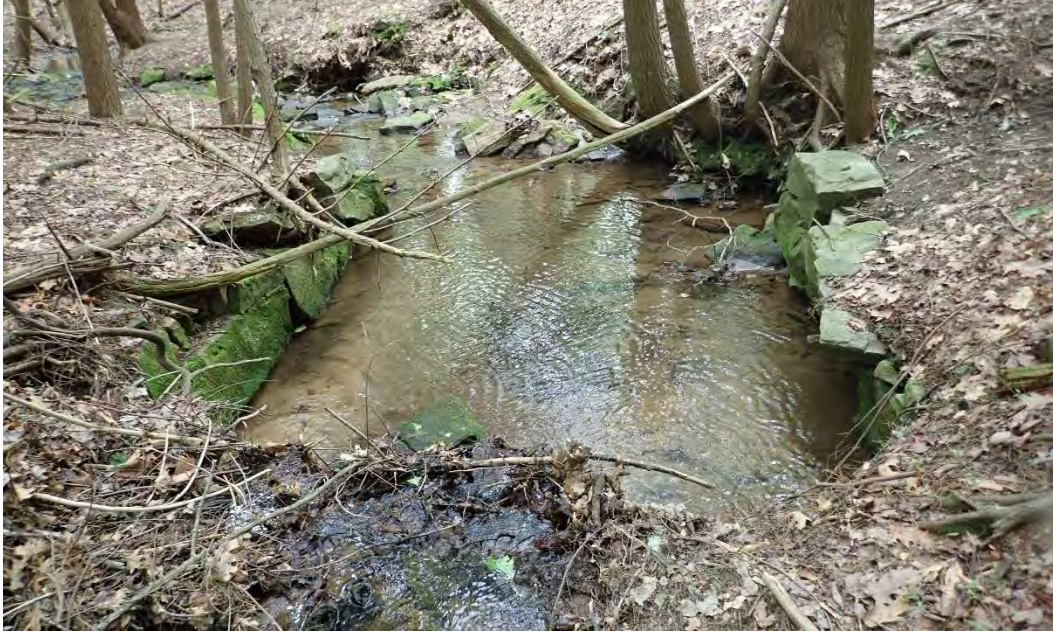
Photo 5. Looking downstream at old bridge abutments made from large, cut boulders.
