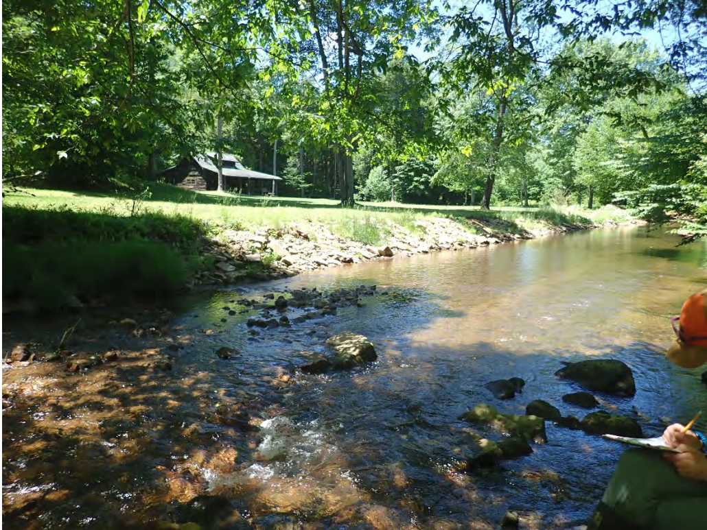
Photo 13. Looking downstream at a camp along segment DG07. Riprap lines the streambank to prevent erosion.
