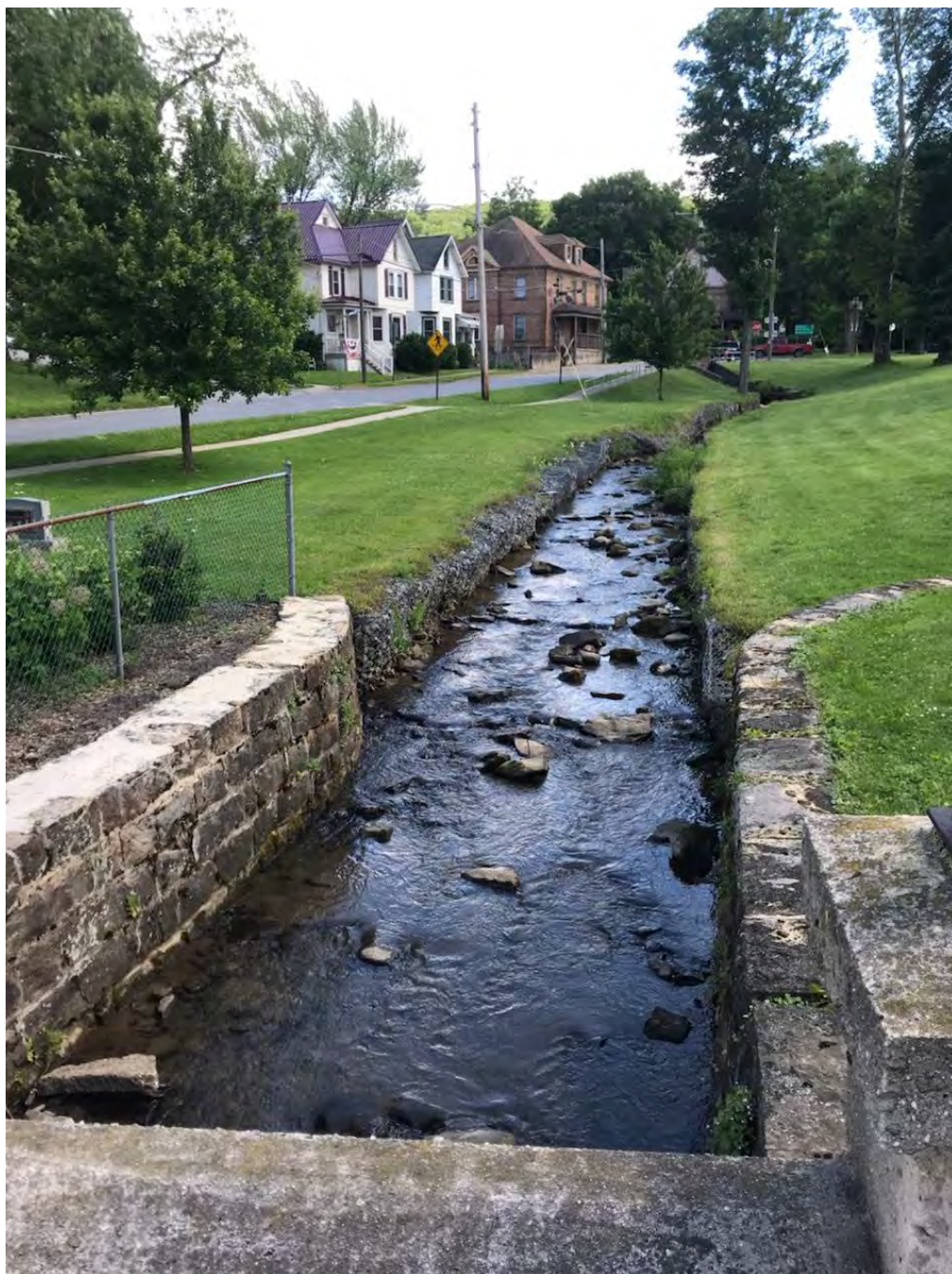
Photo 18. Looking upstream from a footbridge at St. Leo's Catholic School. The stream is impounded with gabion baskets which are falling into the stream channel.
