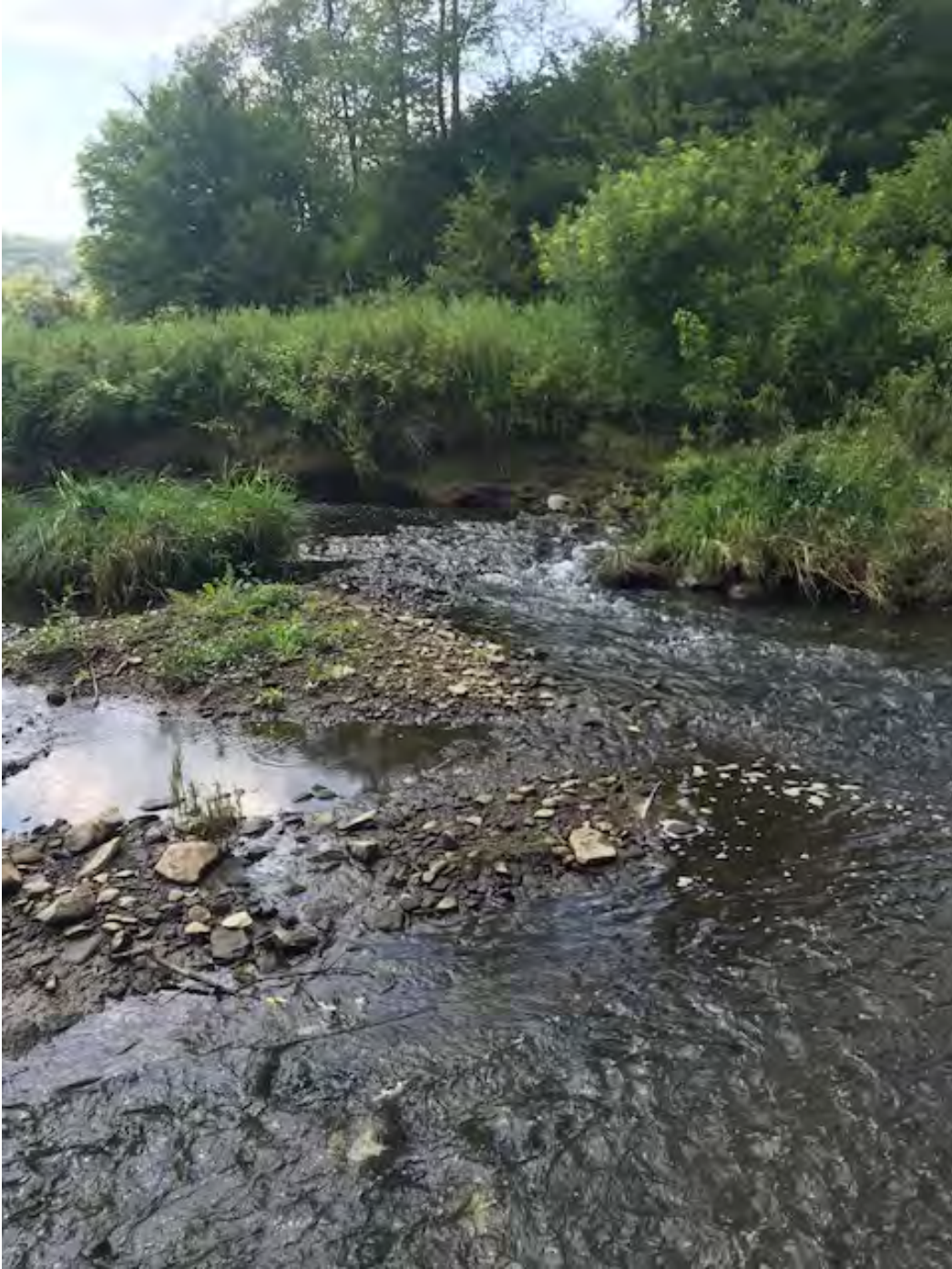
Photo 67. Eroding left bank at the confluence of EC13 and Laurel Run.
