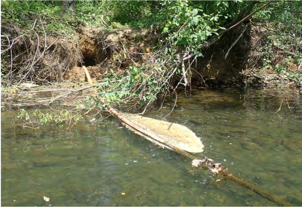
Photo 120. Utility line crossing EC17.
