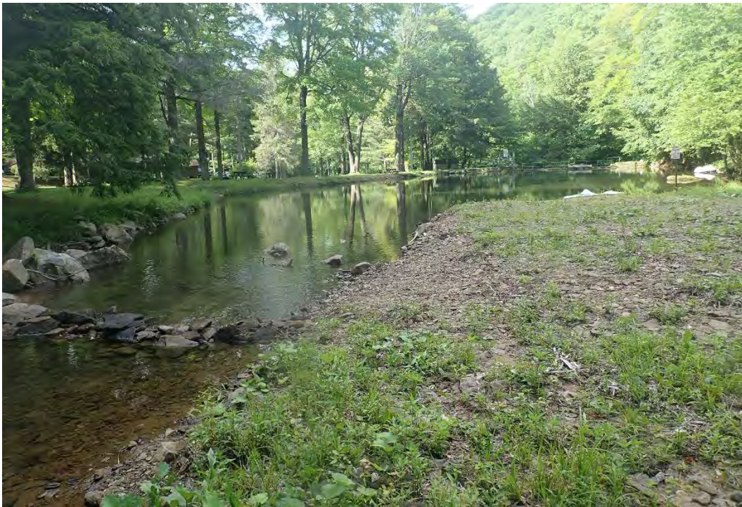
Photo 29. Looking downstream at the Camp Kaelber Dam from Mohan Run.
