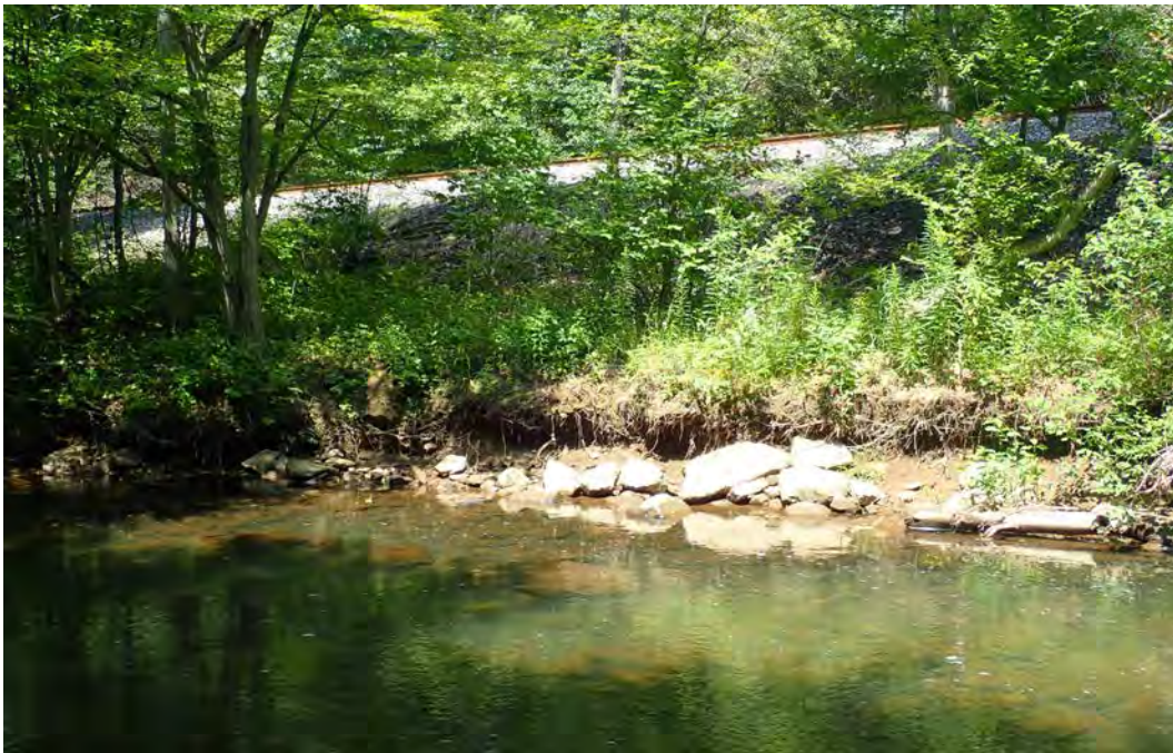
Photo 113. Railroad encroachment in EC16.
