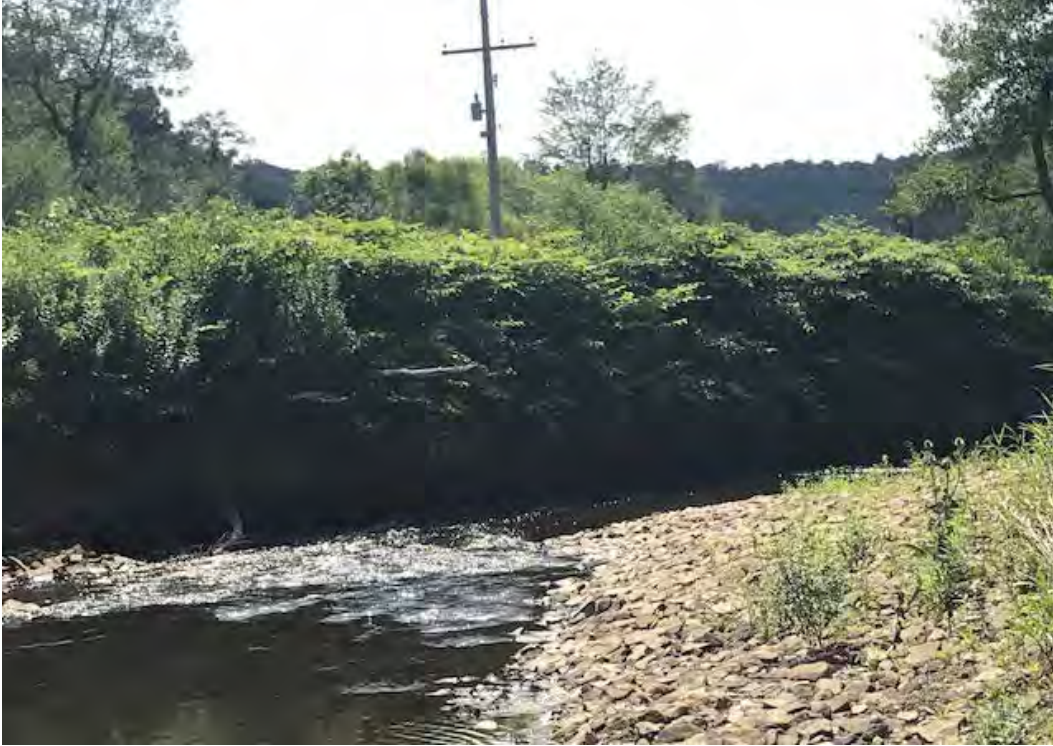
Photo 63. Left bank erosion in EC12 along the powerline right-of-way. Streambank stabilization projects could help protect the electric poles from eroding into the stream channel.
