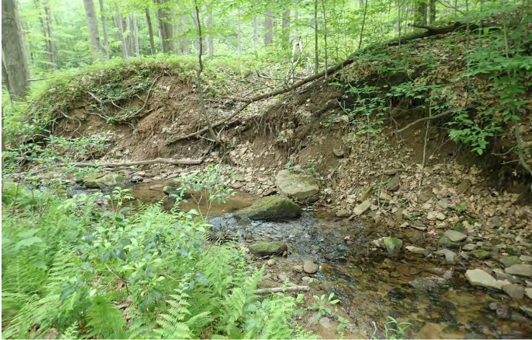
Photo 13. Left bank erosion at the toe of an ATV trail.
