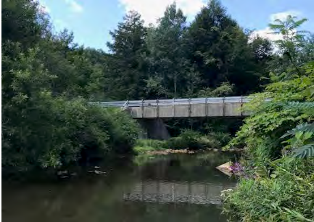
Photo 41. Beginning of segment EC10 looking downstream at the bridge that connects the St. Marys Sewage Treatment Plant to Highway 120.
