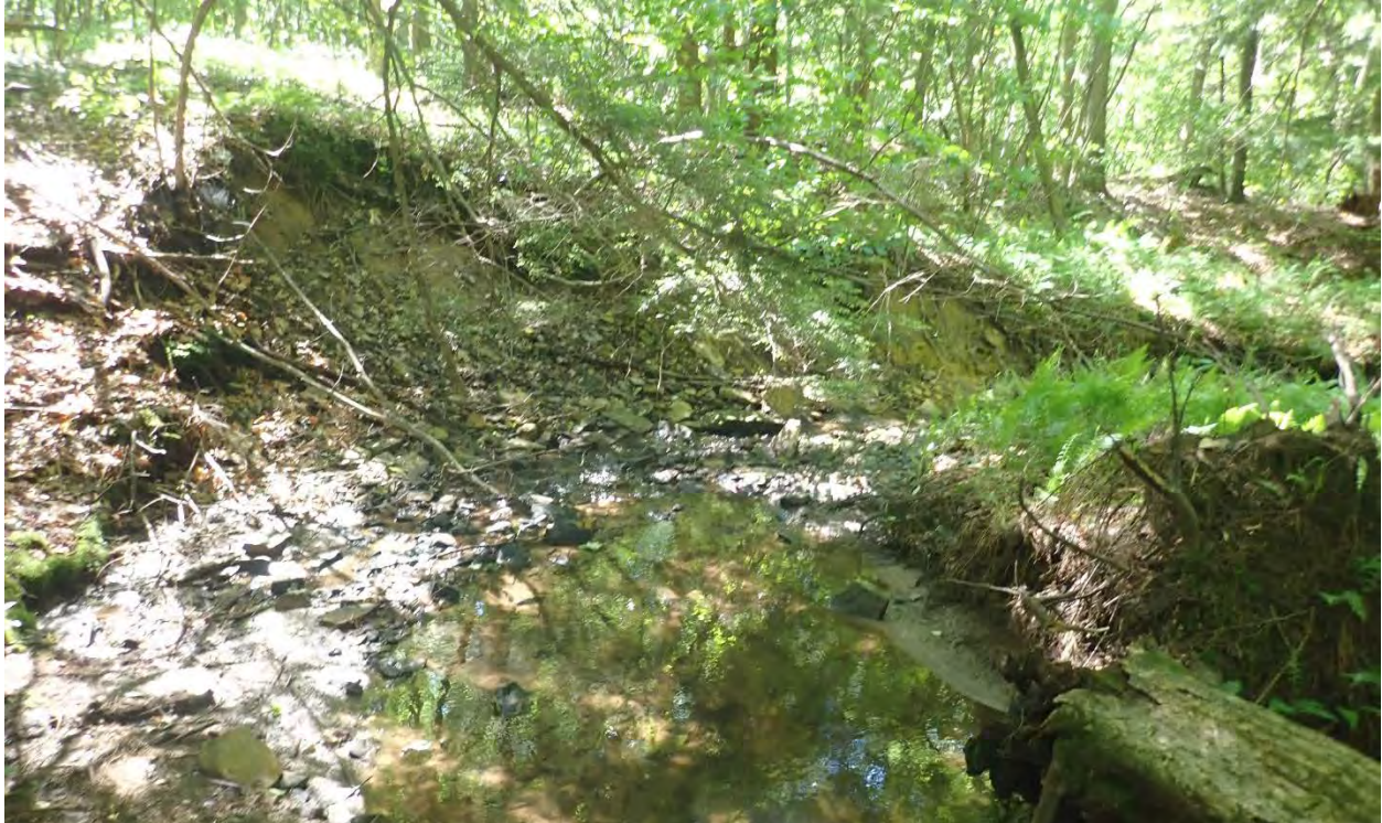
Photo 1. Eroding bank on an outside bend in TC02. Adding large woody debris in this section of the stream would help slow and redirect water to reduce erosion and downstream sedimentation.
