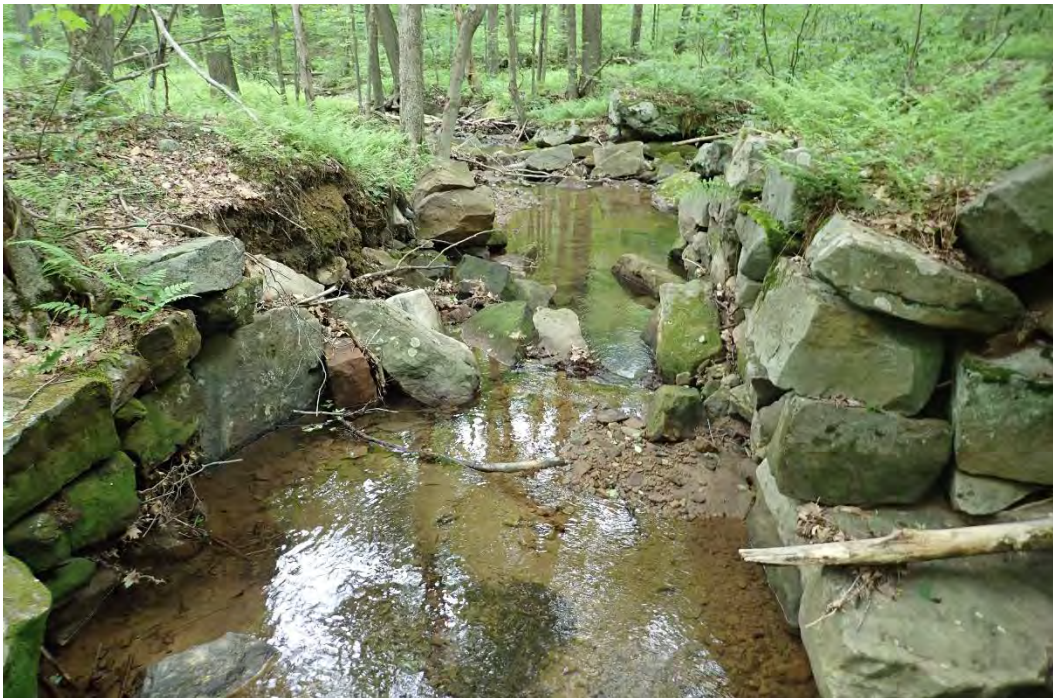
Photo 14. Former bridge abutments made from cut boulders along the stream channel. Some erosion is present on the left bank where the abutments are falling into the stream channel.
