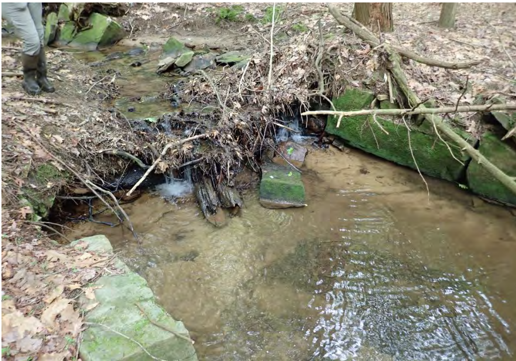
Photo 6. Upstream view of the relic abutments in photo 5. There was an approximately 2ft tall step before the former location of the bridge.
