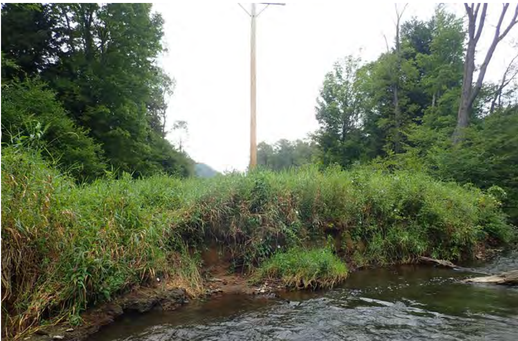
Photo 87. Left bank erosion at the powerline right-of-way crossing in EC14.
