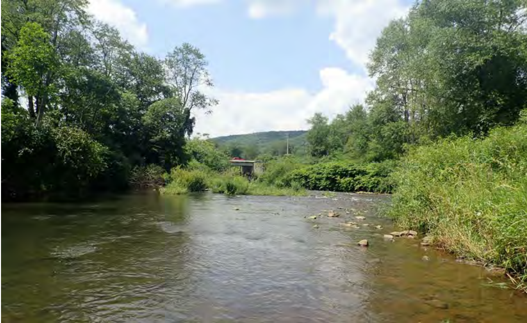
Photo 100. Looking downstream from the beginning of segment EC09. The Bridge Street bridge in Daguscahonda is visible in the background.
