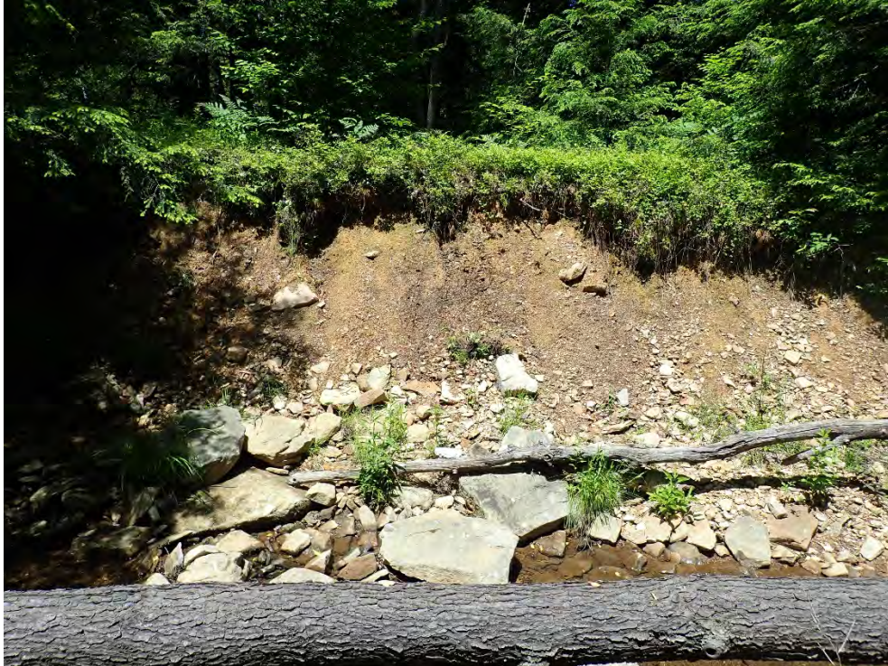
Photo 25. Streambank erosion in LR08 where the powerline right-of-way encroaches on the stream channel.
