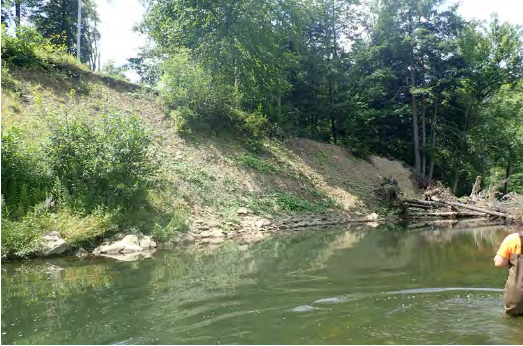
Photo 118. High, eroded left bank in EC17.
