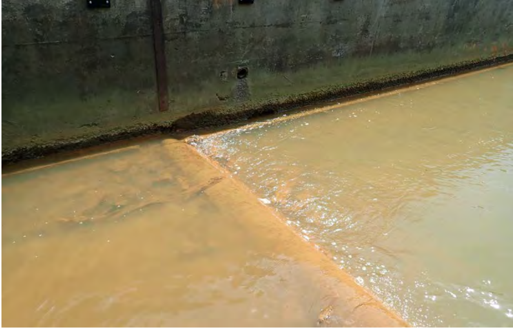
Photo 24. Pipeline laying above the streambed in EC05.
