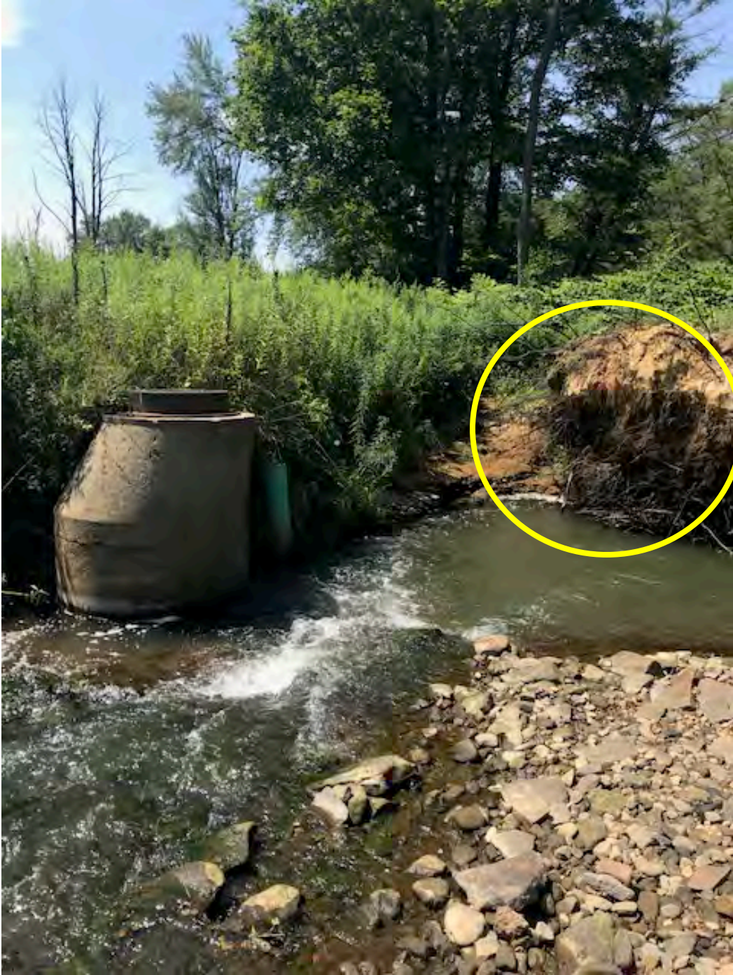
Photo 52. Sewer line manhole lid stack in the stream channel. The manhole stack has rerouted stream water in to the left bank to cause erosion. The erosion caused a tree to uproot (yellow circle).
