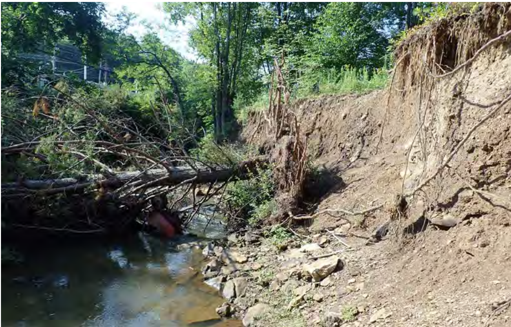
Photo 33. The same eroded streambank from photo 32.
