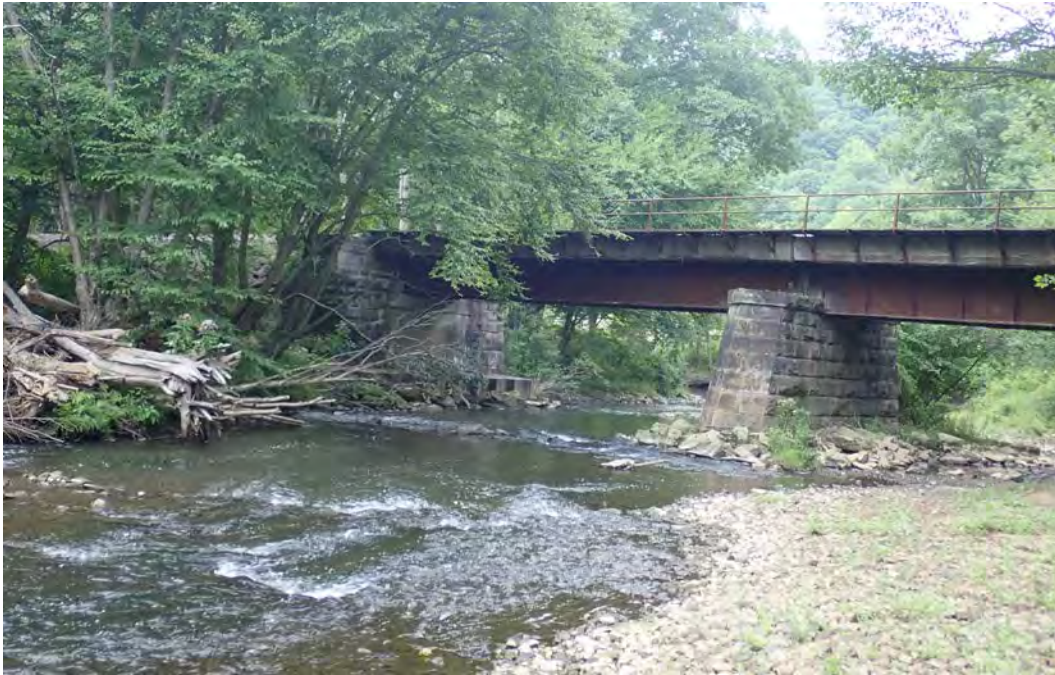
Photo 129. Railroad bridge over segment EC18.
