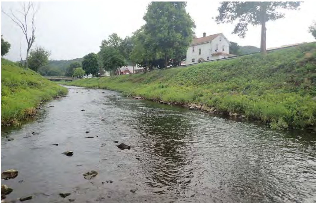
Photo 149. Channelized portion of EC19 looking upstream at the Depot Street bridge.
