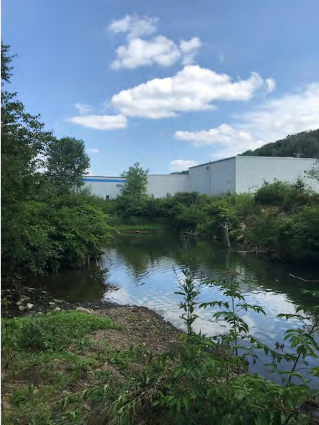
Photo 57. Looking upstream at the Custom Industrial Processing building within the floodplain of EC12. Restoring trees in the riparian area between the building and the stream channel is encouraged to prevent the parking lot from eventually eroding into the stream channel.
