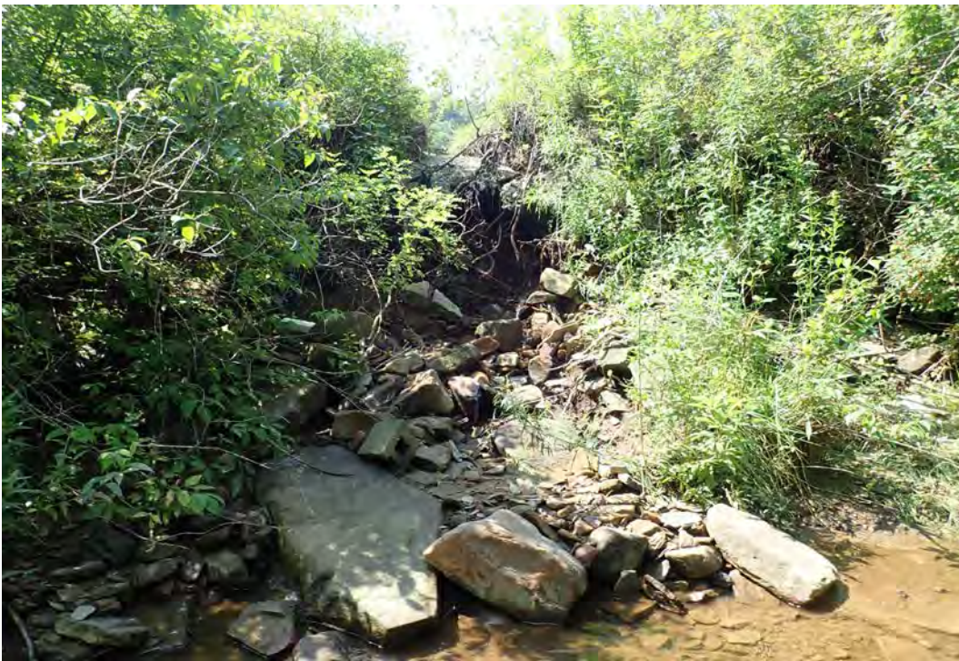
Photo 37. Erosion from stormwater overflow off the Keystone Powdered Metal parking lot in EC07.
