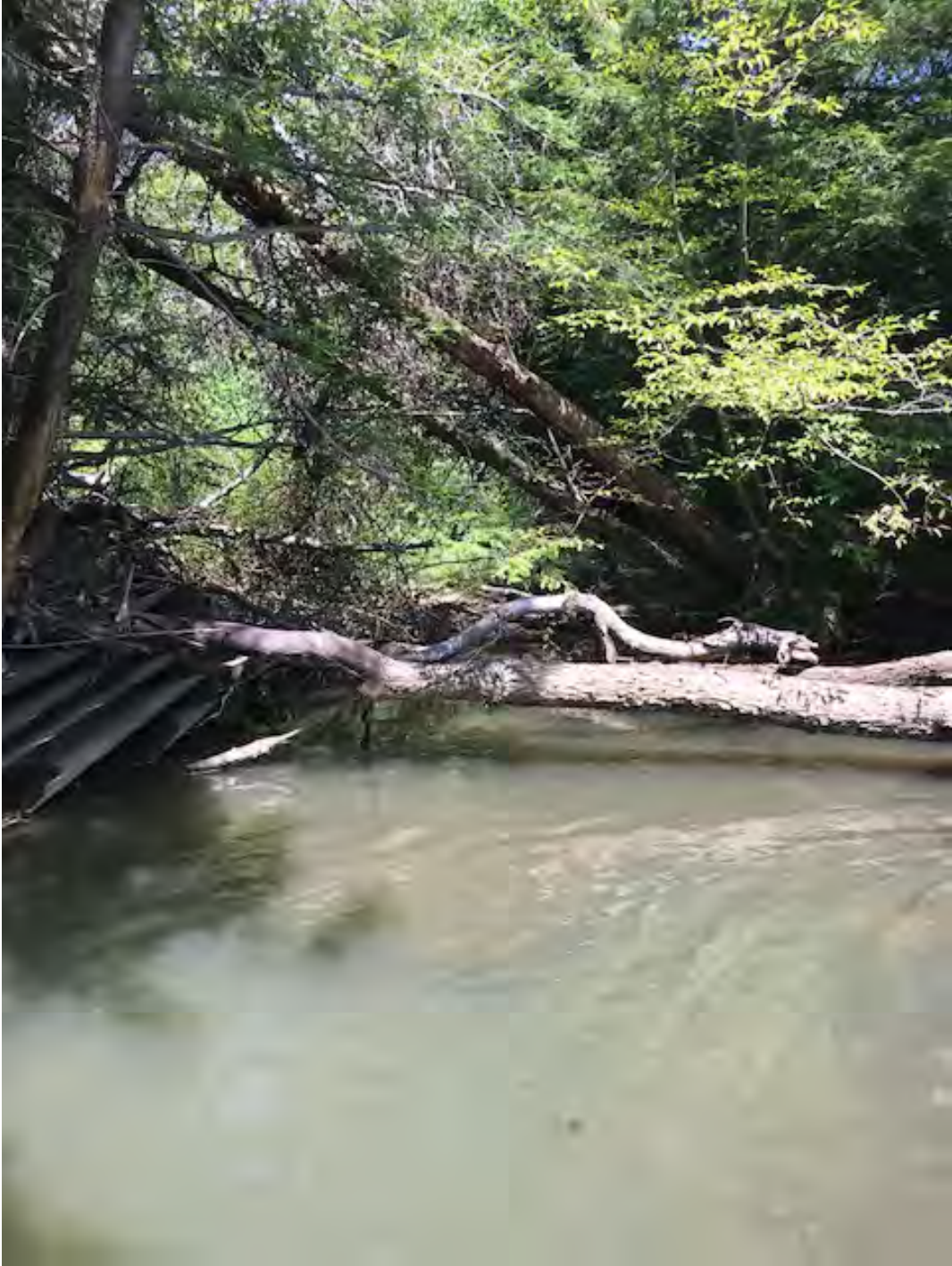
Photo 50. End of EC10 looking downstream at the confluence with Silver Run and a debris jam.
