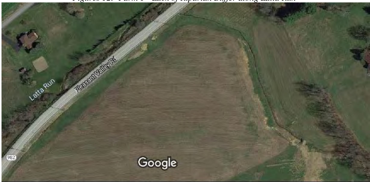
Figures 12: Farm 1 - Lack of Riparian Buffer along Latta Run
