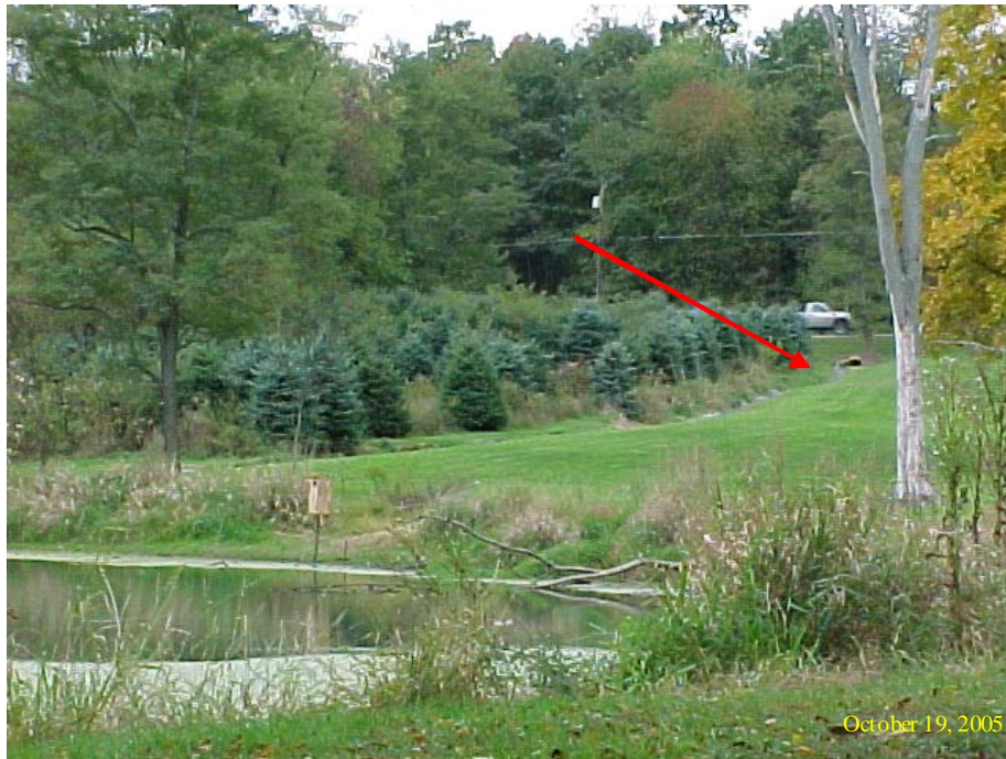
Route 388 culvert carrying stormwater through a series of residential ponds.
