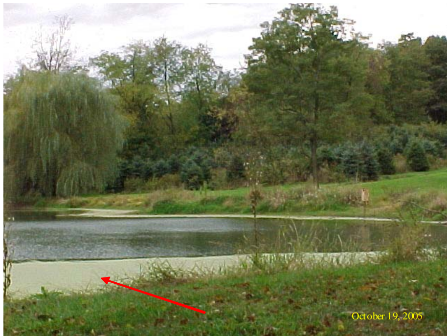
Algal growth on the surface of the pond can be one indicator of nutrient enrichment. Keeping the stormwater conveyance channel vegetated assists with nutrient uptake and removal of non-point source pollutants.
