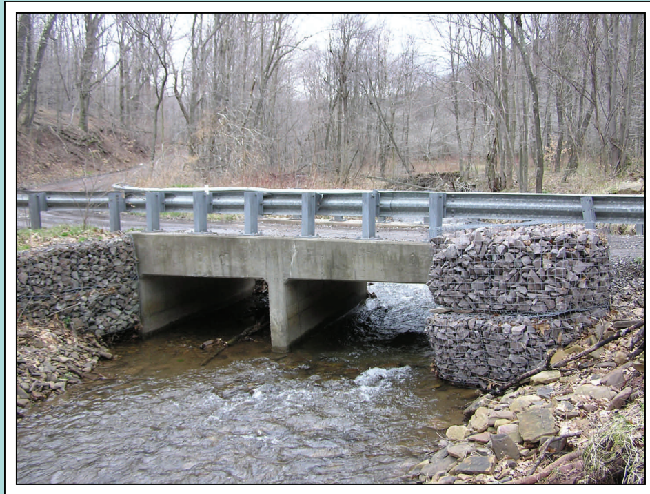
Upstream view of Shirley Hollow Road bridge, above sample site MI-5.
