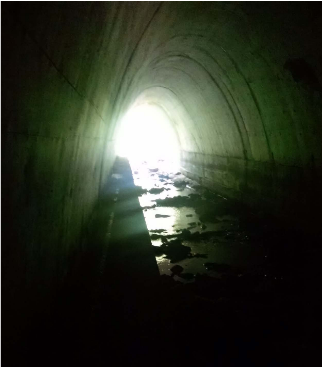
Figure 66: Inside Culvert under 81 near Laurel Run #2 Dam (Photo 62)
