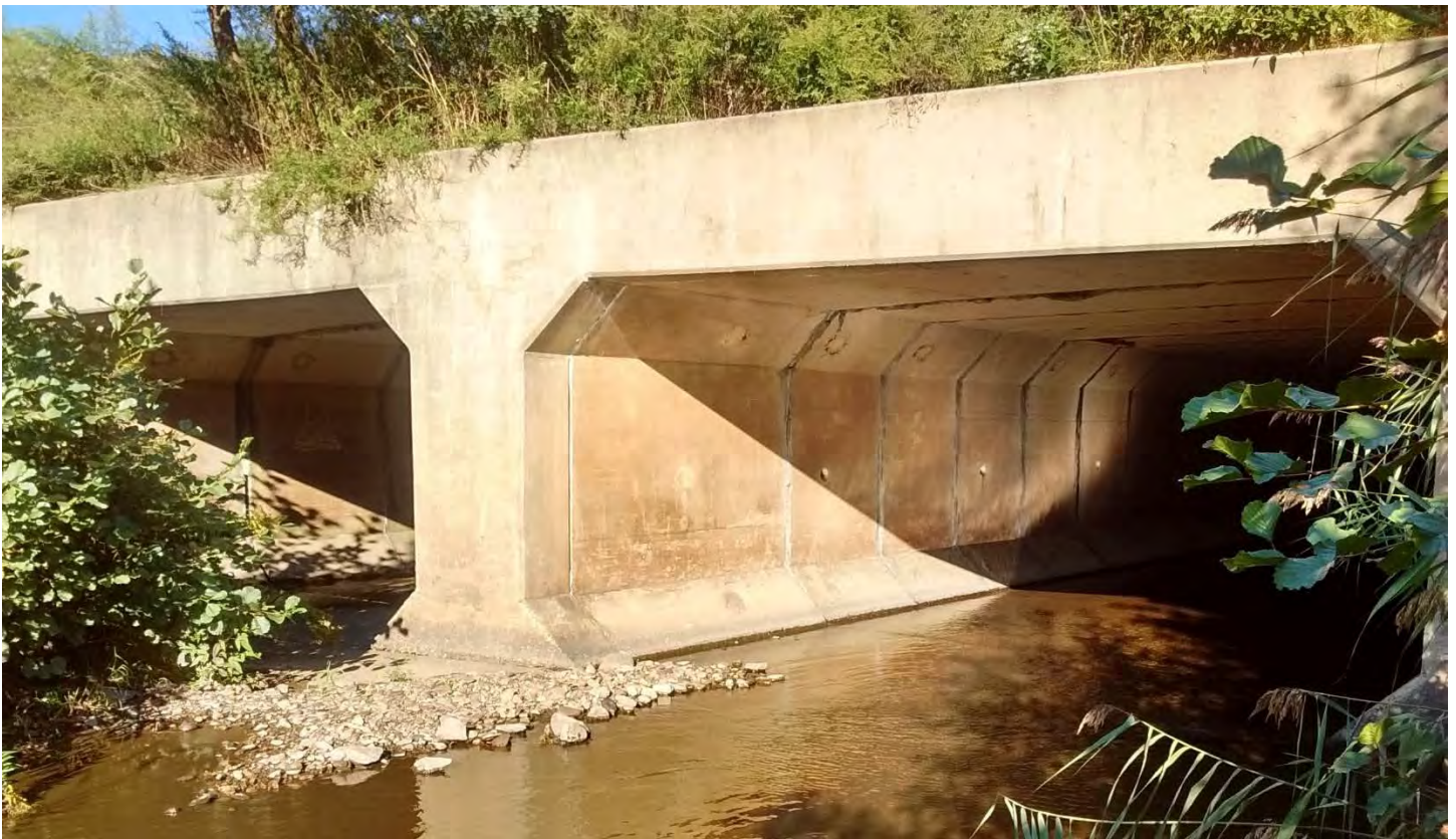
Figure 60: Culvert #2 Inlet (Photo 56)
