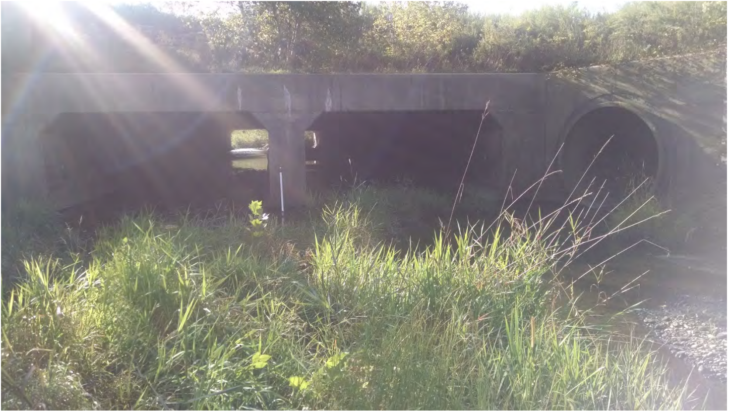
Figure 61: Culvert #2 Outlet (Photo 57)
