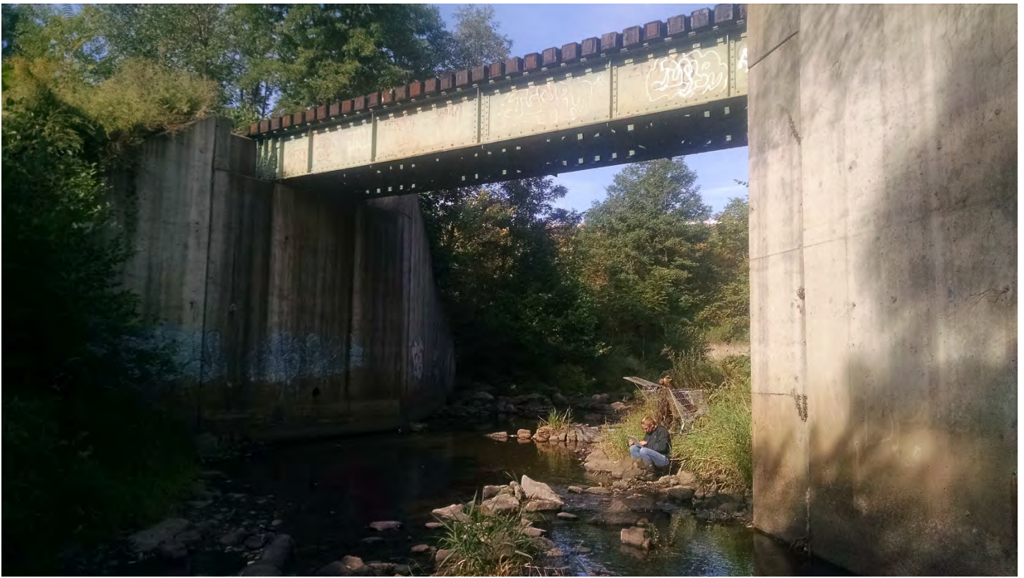
Figure 64: Train Crossing Inlet (Photo 60)
