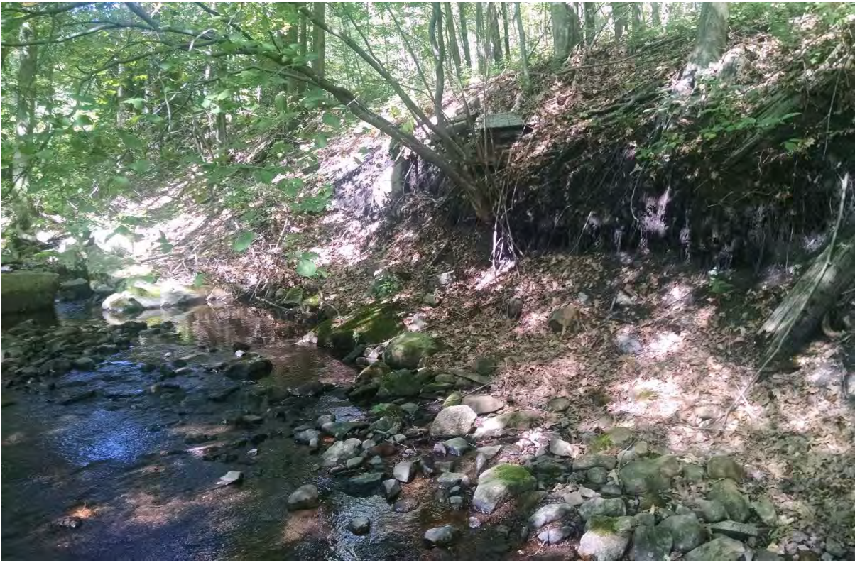
Figure 52: LR13 Upstream (Photo 48)
