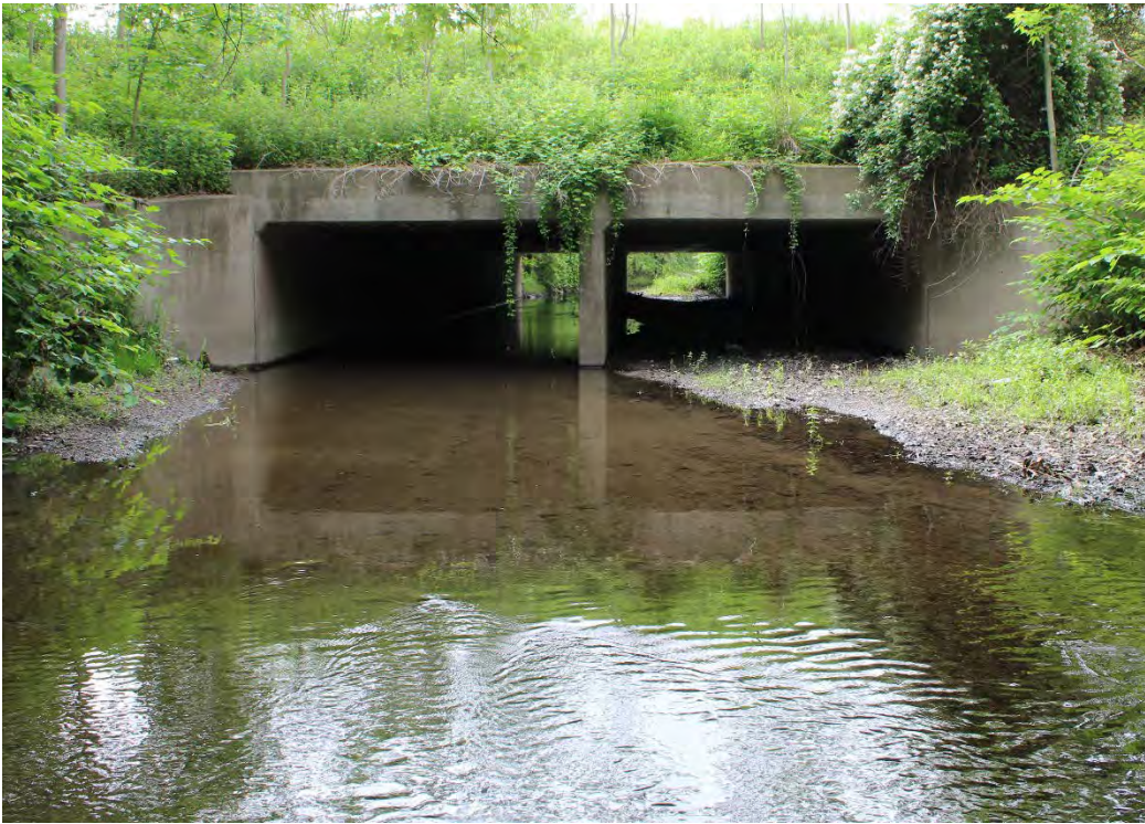
Figure 7: LR1 Upstream (Photo 2)
