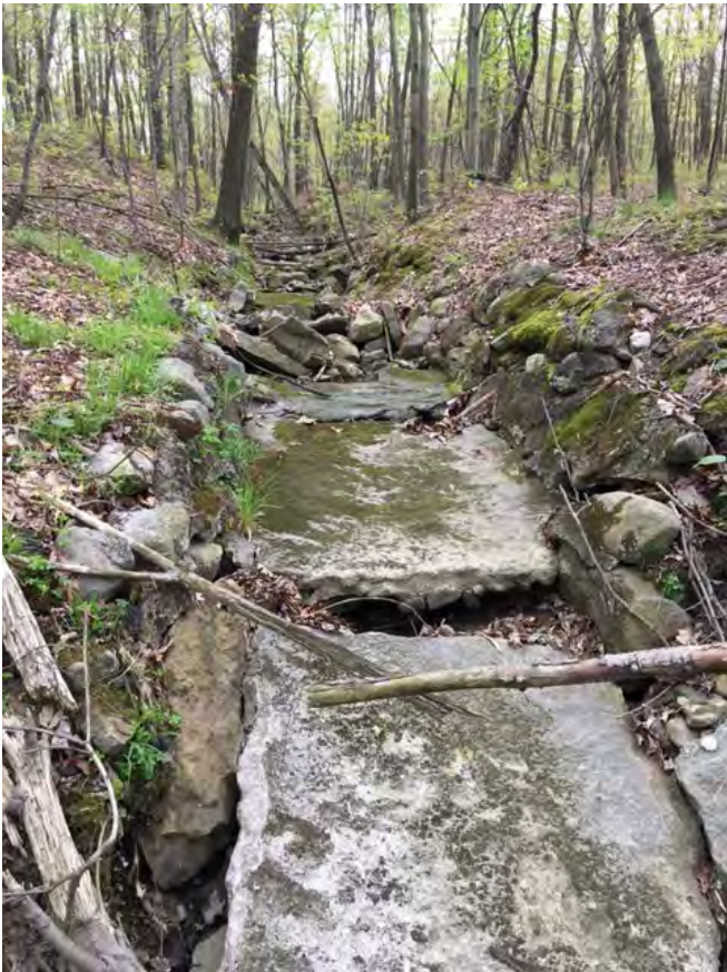
Figure 27: CB3 Upstream (Photo 22)
