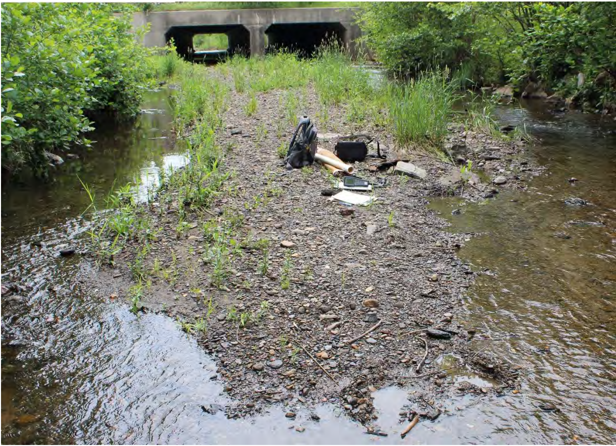
Figure 9: LR2 Upstream (Photo 4)
