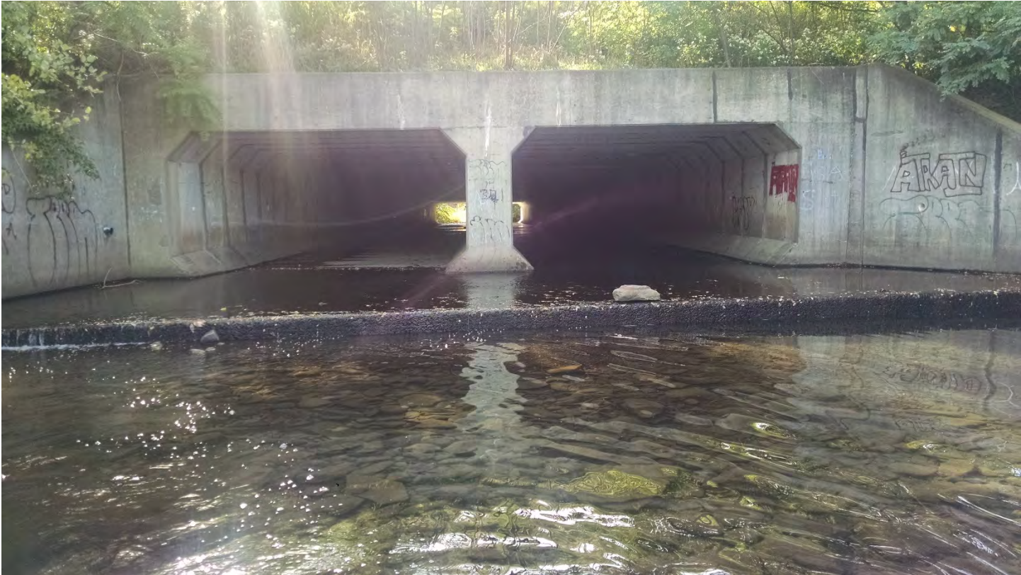
Figure 63: Culvert #3 Outlet (Photo 59)
