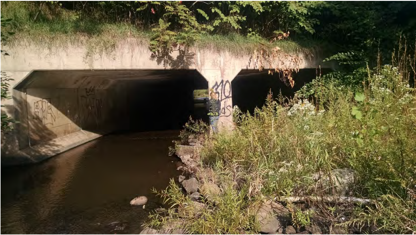
Figure 62: Culvert #3 Inlet (Photo 58)
