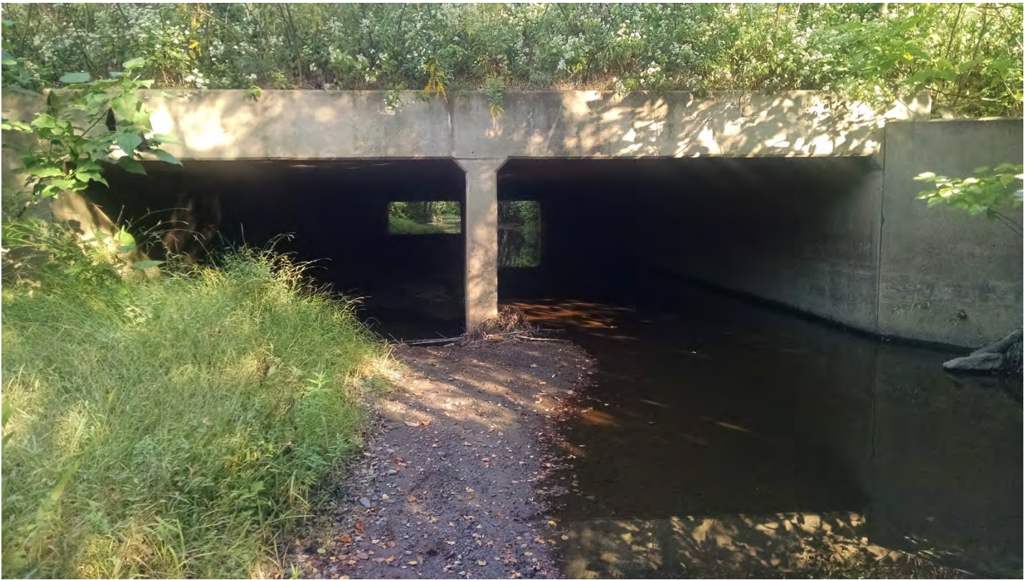
Figure 58: Culvert #1 Inlet (Photo 54)
