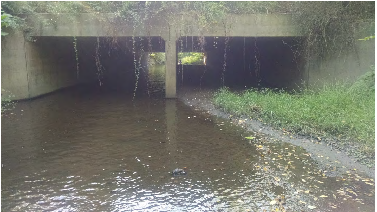
Figure 59: Culvert #1 Outlet (Photo 55)
