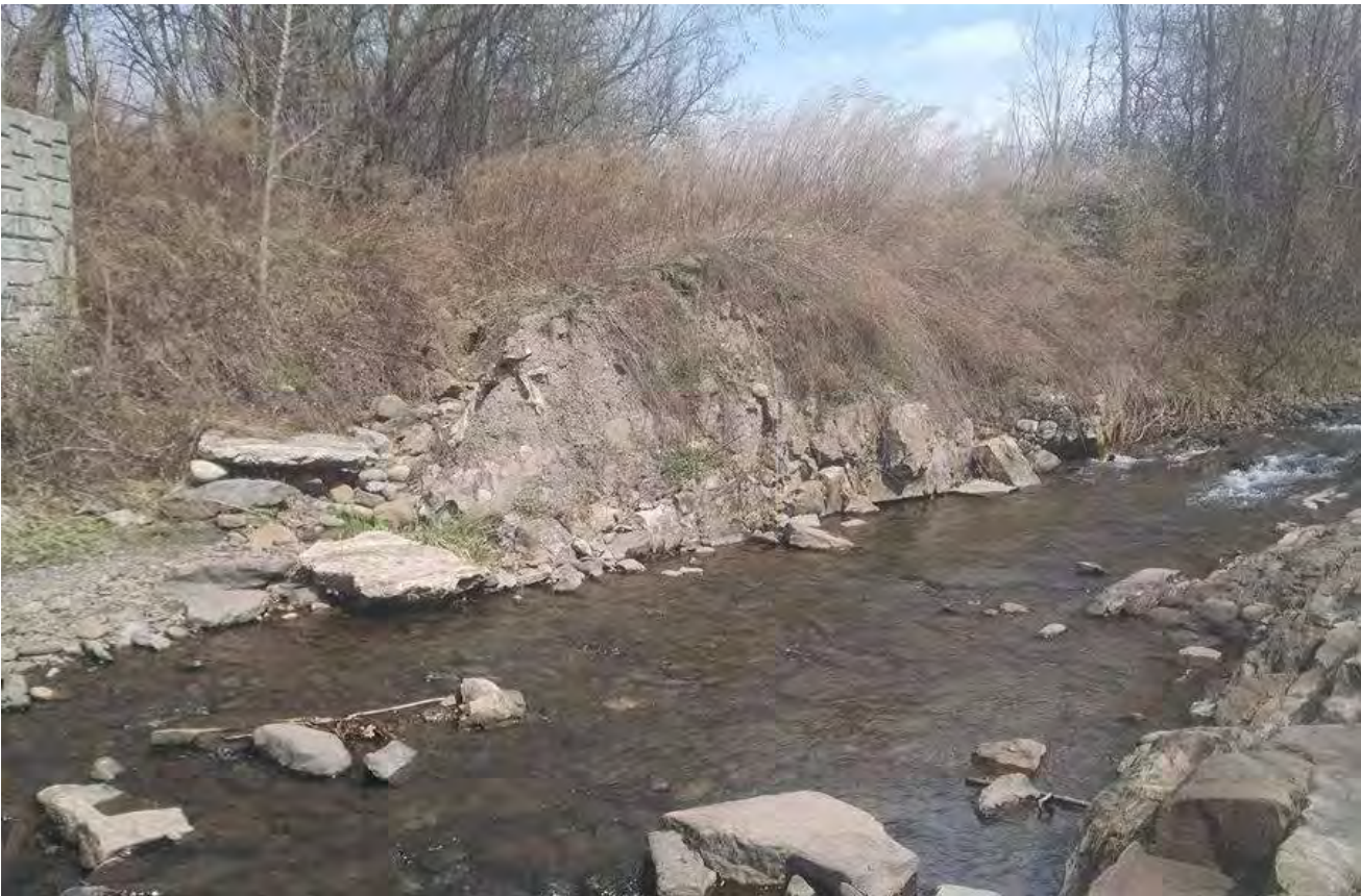
Figure 16: Erosion near LR4 (Photo 11)
