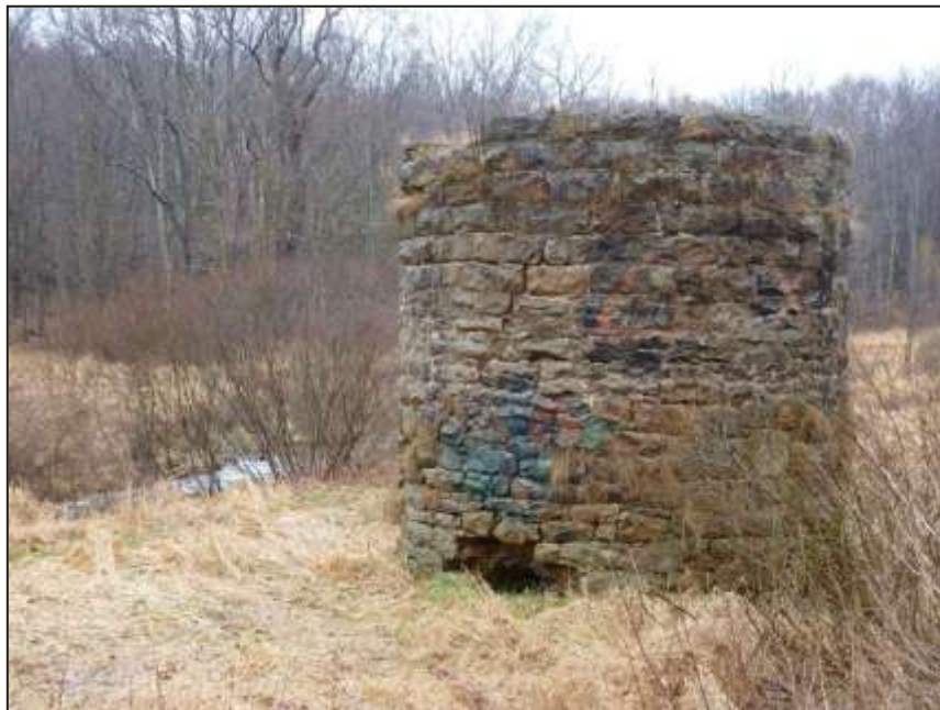
Figure 53. The remains of a round structure along Little Paint Creek said to float coal and separate it from rock. Photo by Melissa Reckner
