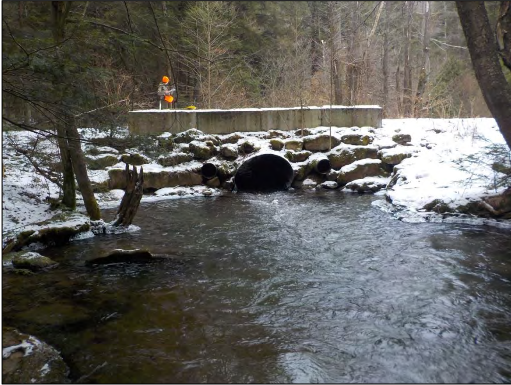
Barrier 6: exhibits “fire hose effect” scour pool at its outlet
