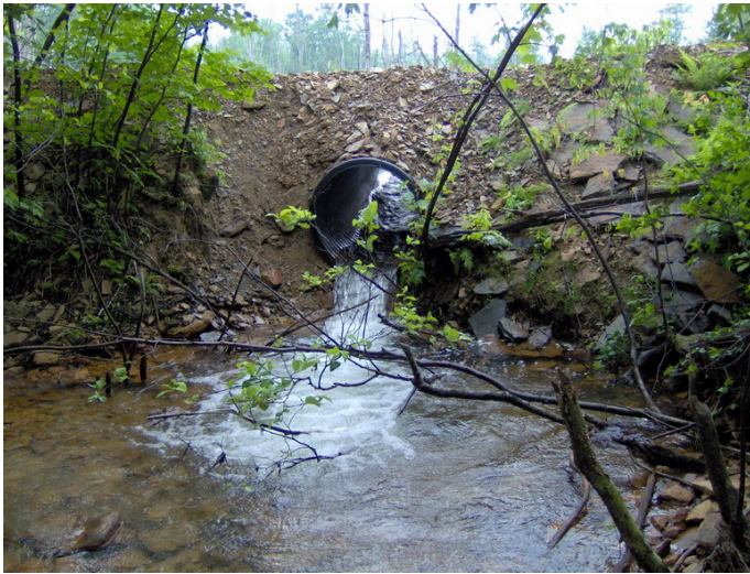
Culvert from dirt road crossing
