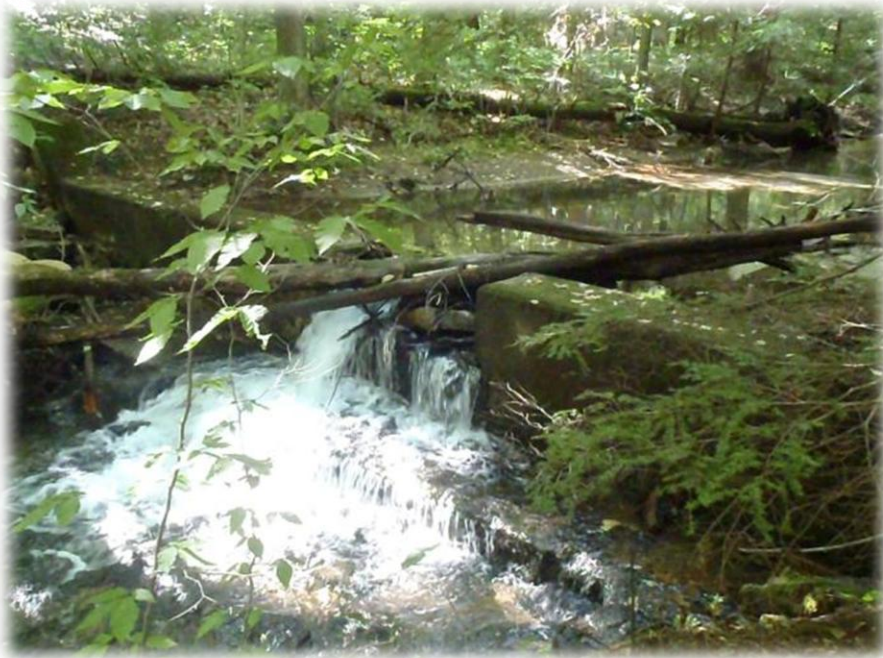
Figure 43: A concrete weir on Alwines Creek. This structure prevented wild rainbow trout from accessing the headwaters of this stream.
