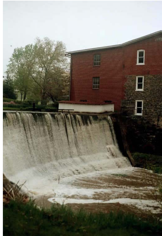
Anthony's Feed Mill Dam on Jackson Creek
