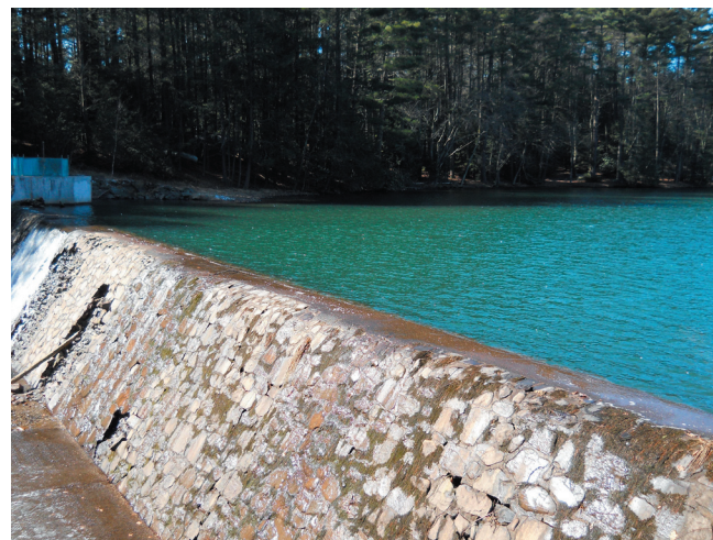
Crawford Lake Dam on the Paradise Creek
