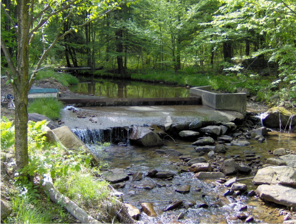
Dam in stream for Westover Municipal Authority
