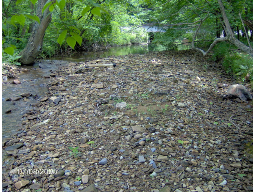
Gravel bar below railroad bridge
