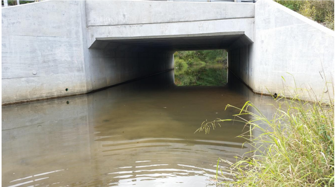
Figure D-2: SL1 looking downstream at SR 255 Bridge
