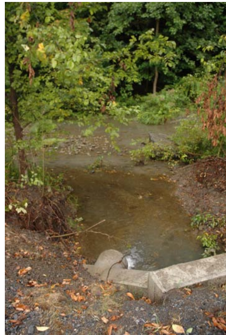
Figure 12 Storm water outfall at Bedford Springs hotel
