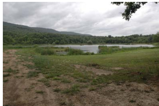
Figure 16 Constructed wetland pond near Shobers Run Lane
