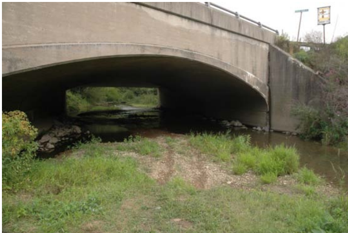
Figure 4 Route 30 bridge at mouth of Shobers
