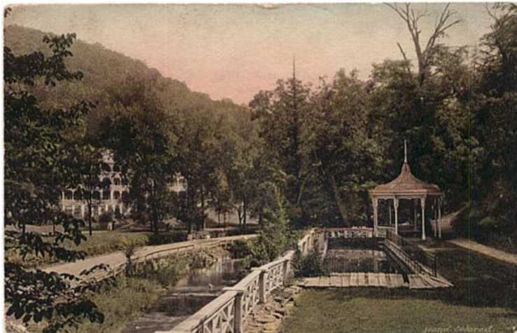
Figure 2 Shobers Run view looking downstream from colonnade
