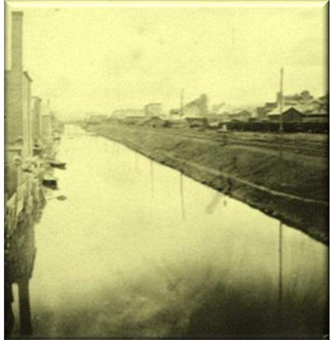
Figure 2-45 Wyoming Canal from South Street Bridge looking North along what would now be Wilkes-Barre Boulevard
