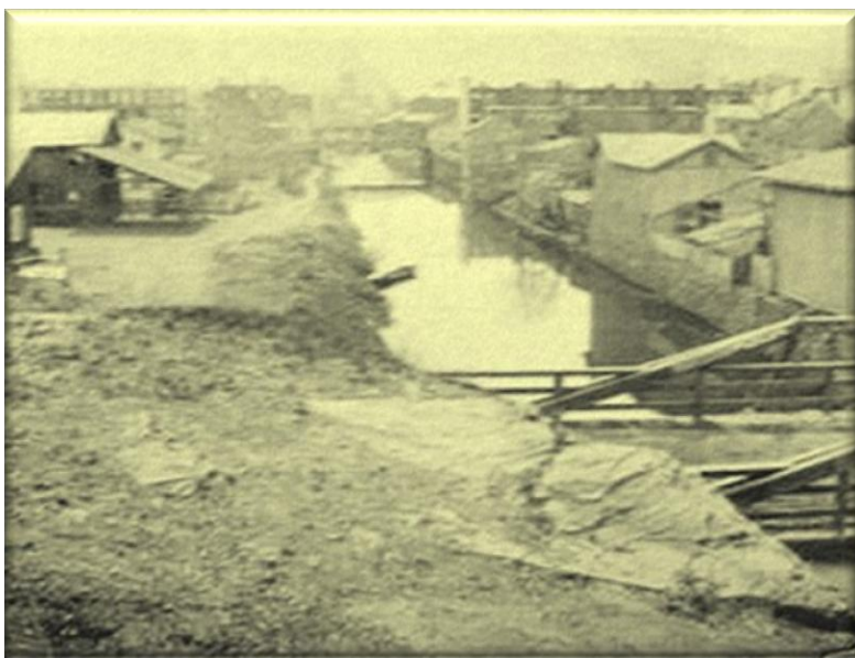
Figure 2-44 Wyoming Canal through Redoubt Bluff in Wilkes-Barre
