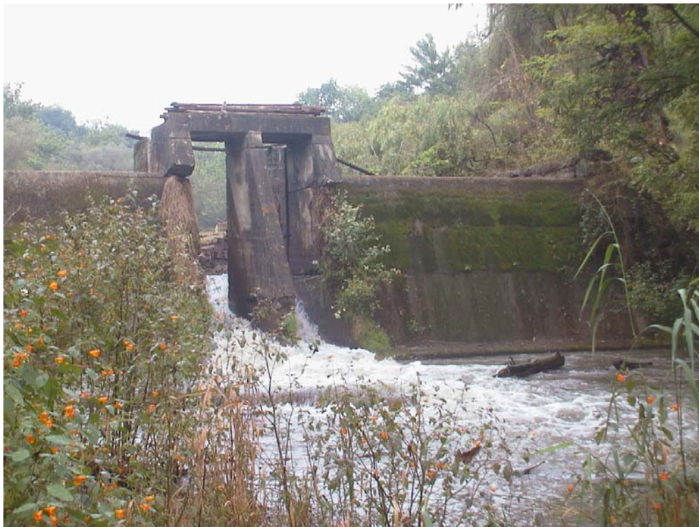
Photo 2: Sediment laden water being released from Reedsville Milling Company Dam with all boards removed
