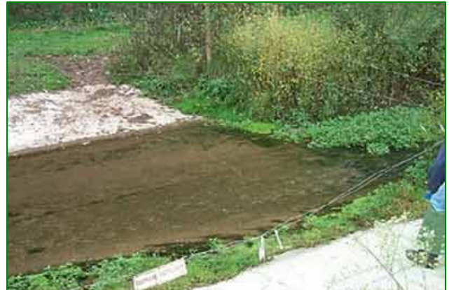
Stabilized crossing at TECR 03
