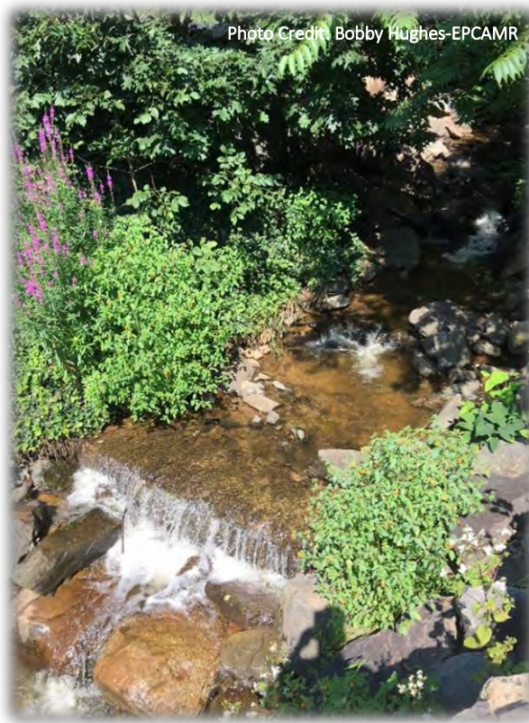
Figure 9. Wildcat Falls, unnamed tributary to Toby Creek flowing over concrete encased sewer line
