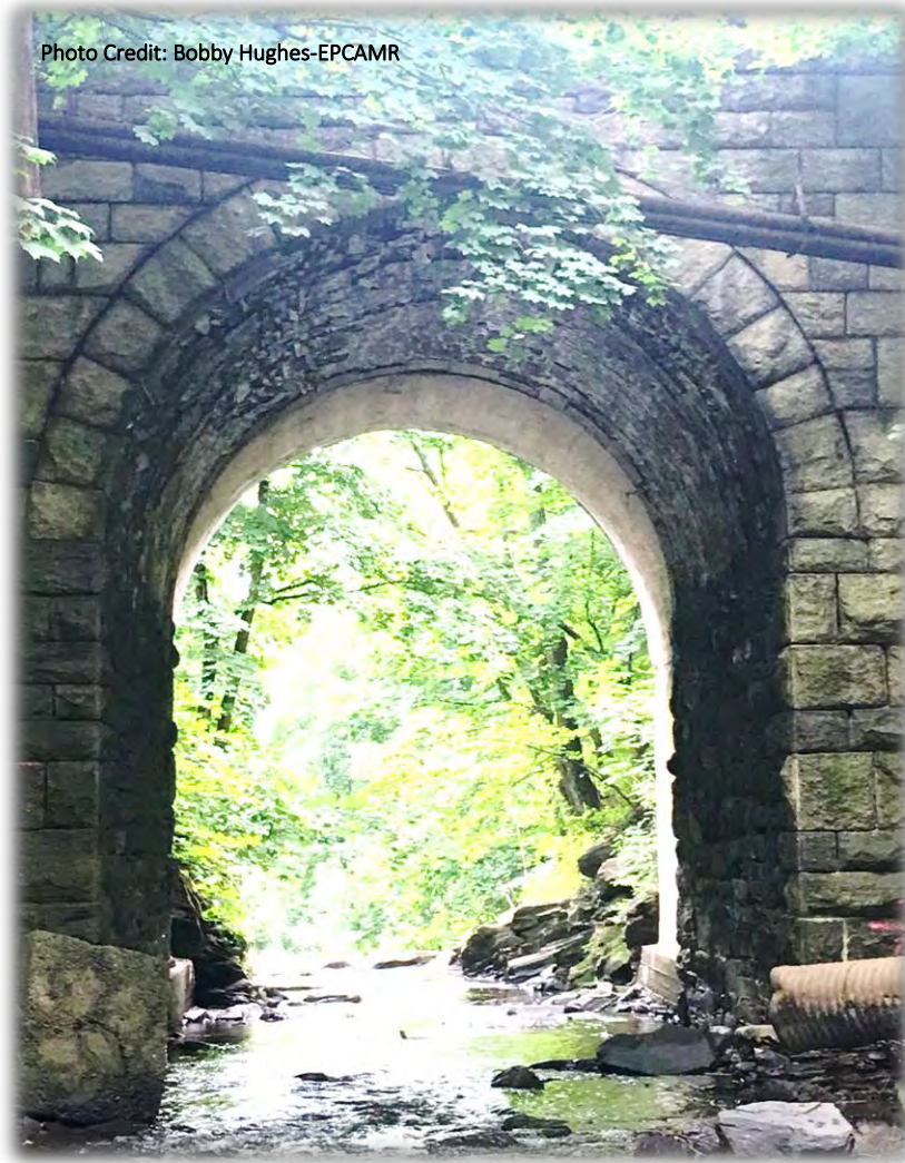
Figure 15. Toby Creek flows downstream through the Stone Arch Bridge over Harris Hill Road
