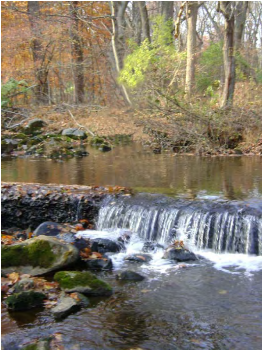
Figure 17. Looking upstream at upper dam on West Branch Crum Creek.
