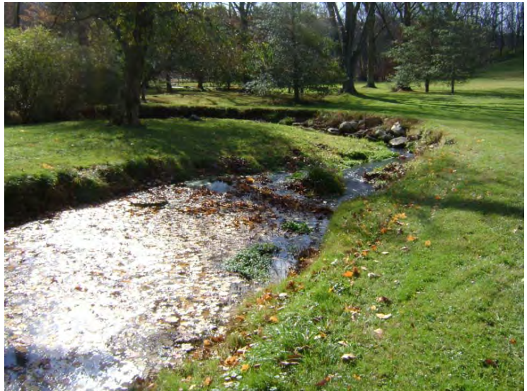
Figure 16. Example of mowing to the top bank along the West Branch.
