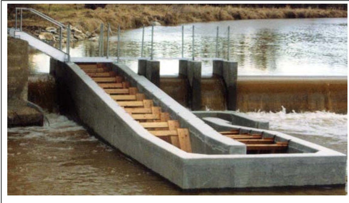
Figure 24. Picture of a typical fish ladder
