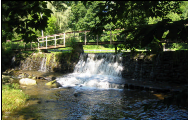
Figure 6. Looking upstream at Mensch Mill Dam
