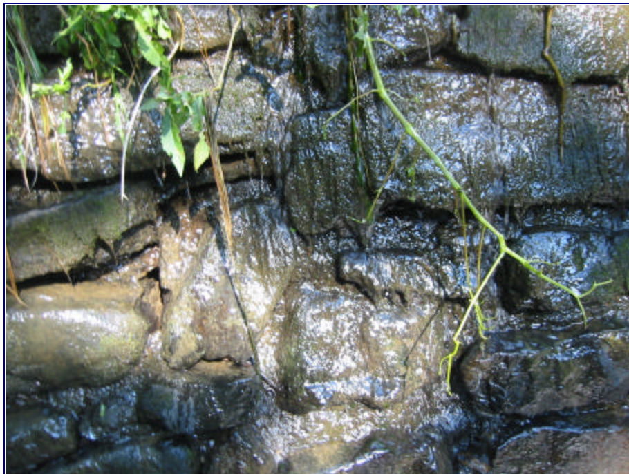
Figure 9. Close-up of downstream masonry face
