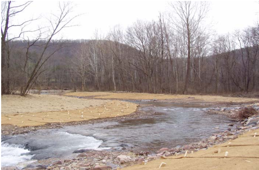
Figure 12. Stream improvement devices stabilize the stream, preventing severe bank erosion behind the Brown home.
