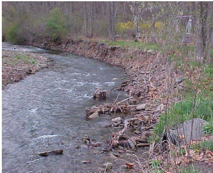
Figure 16: Wallace Run before restoration
