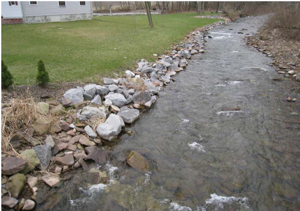
Figure 4. When riparian vegetation is removed, home owners immediately begin trying to stabilize the bank with rock.
