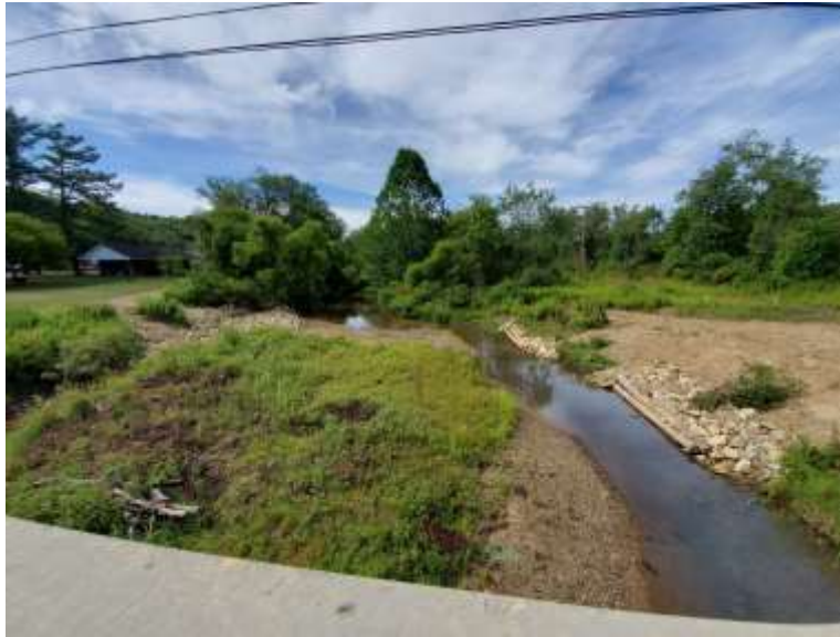
Upstream nearly a month after construction 8/21/20
