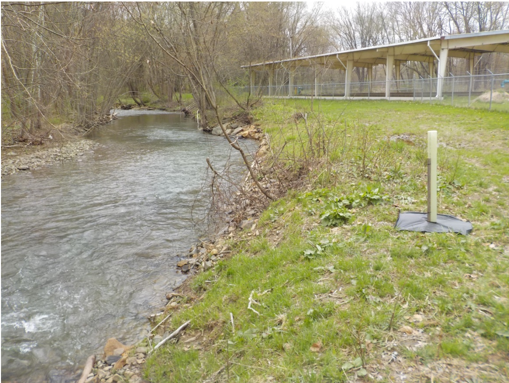
AFTER: A log-framed stone deflector (right foreground) and modified mudsill (right background) provide bank stabilization and improve habitat diversity and cover for fish
