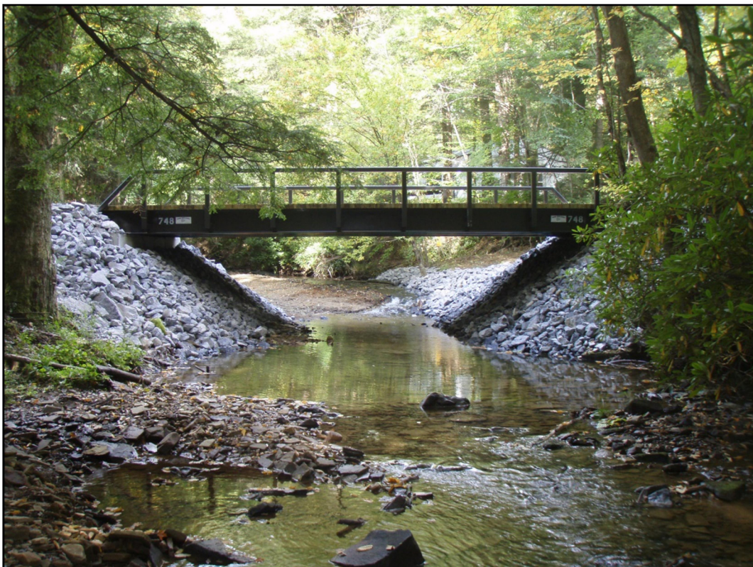
Forest Road 156 Outlet AFTER restoration
