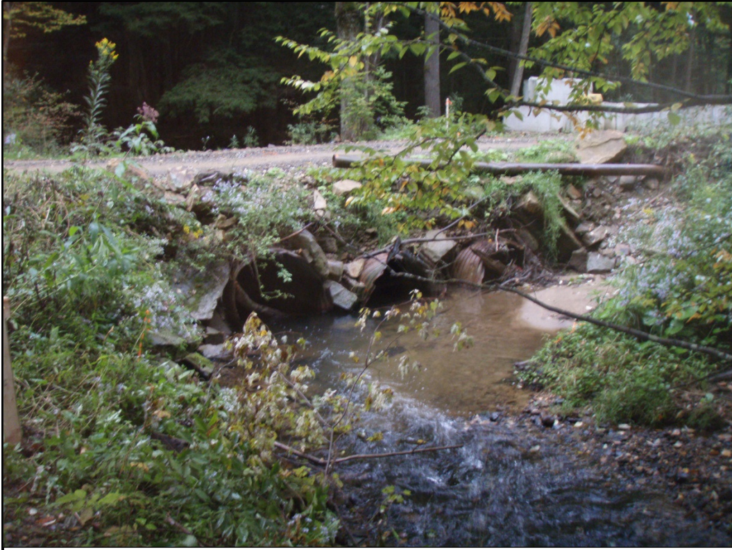
Forest Road 156 culverts inlet BEFORE restoration
