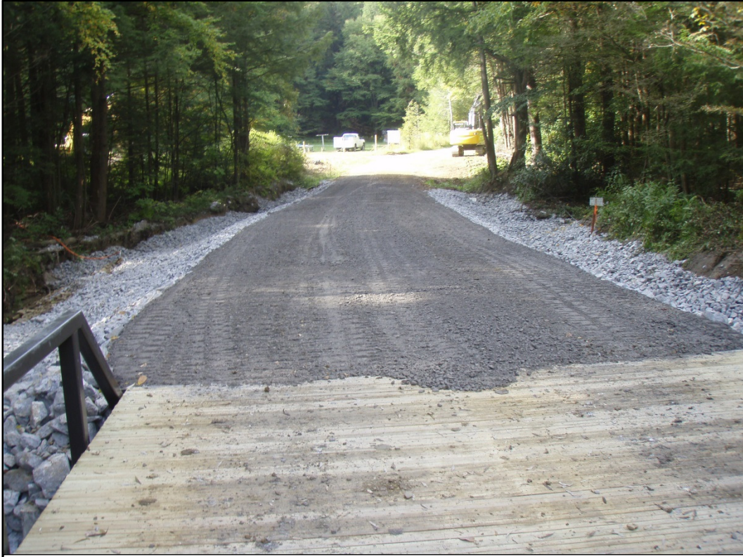
Forest Road 156 AFTER resurfacing with DSA and limestone ditch lining
