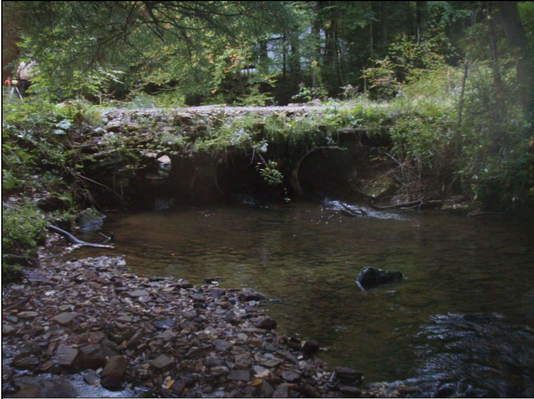
Forest Road 156 culverts outlet BEFORE restoration
