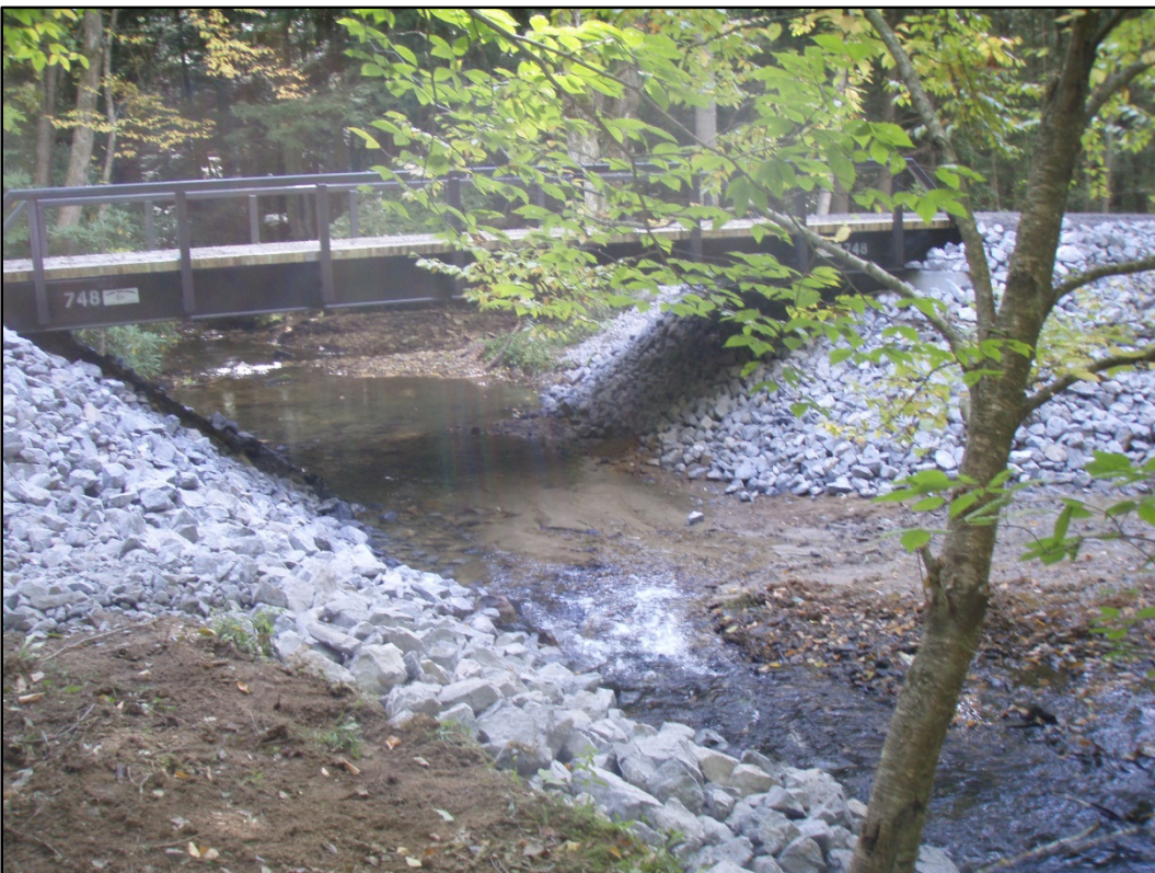
Forest Road 156 Inlet AFTER restoration
