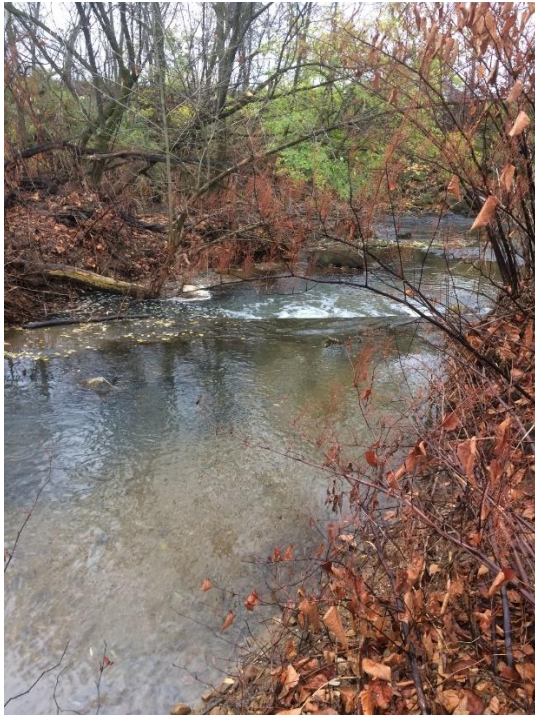
Image 1: Looking downstream at the dam
