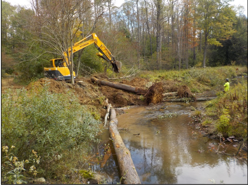
Photo 4. Rootwad installation. September, 2017.
