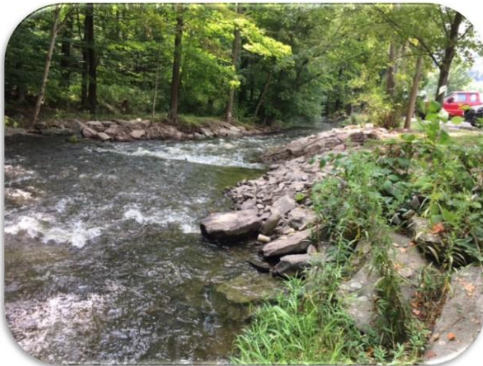
These photos show the addition of rip-rap on both banks.
