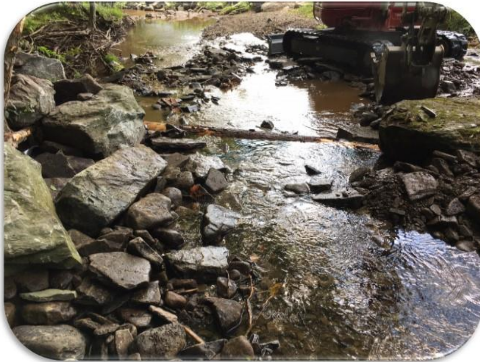
The above photo shows the second of the three log vanes installed also at low flow conditions.
