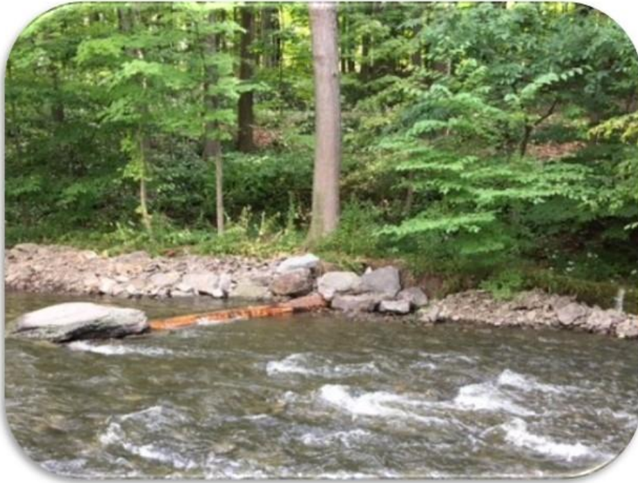
These photos show the addition of rip-rap on both banks.
