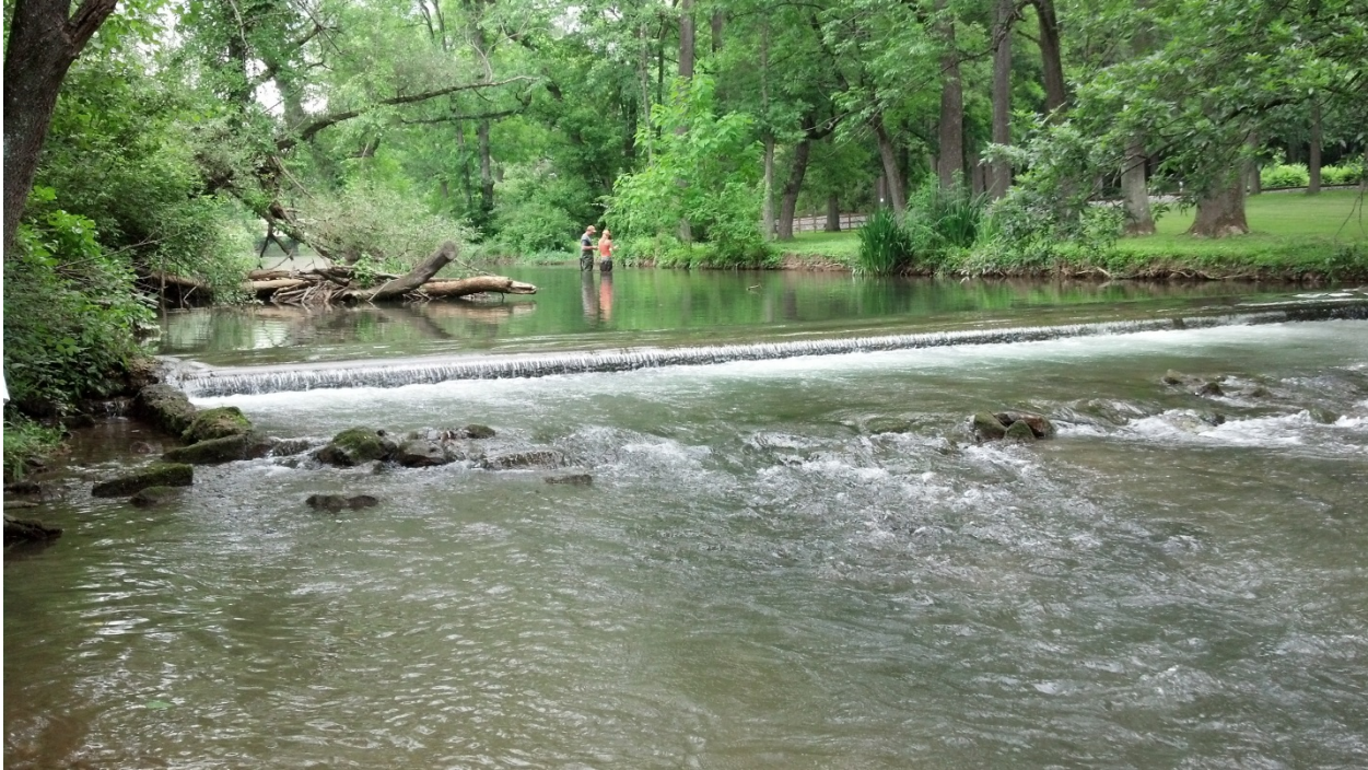
Before project: the dam on Monocacy Creek obstructing flow and degrading habitat.
