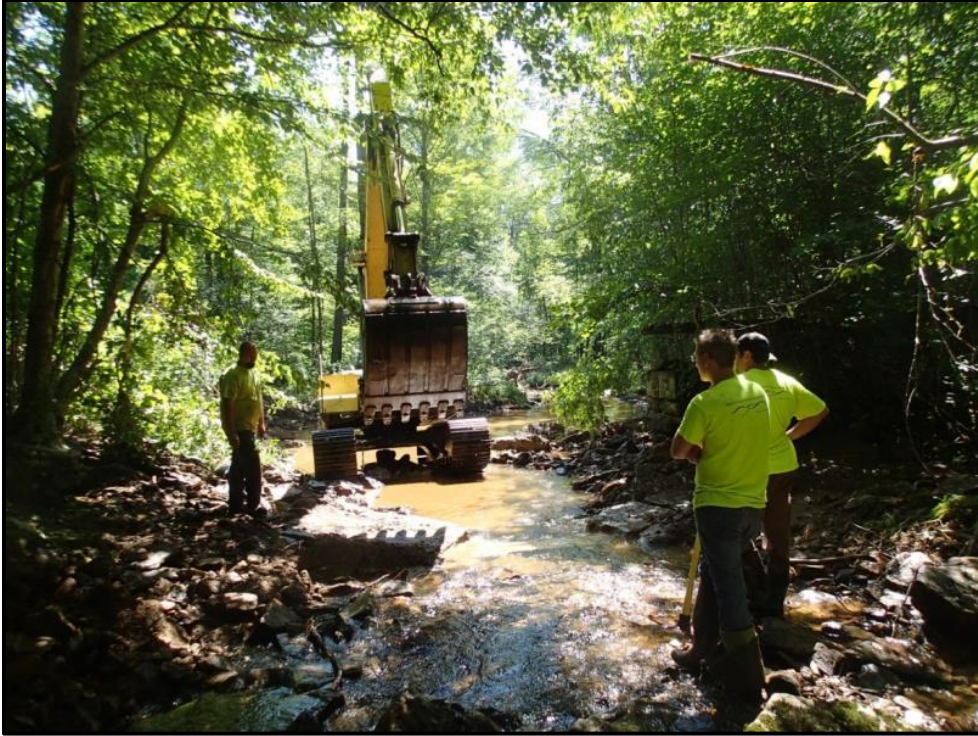
Figure 8 - Installing the rock cross vane.
