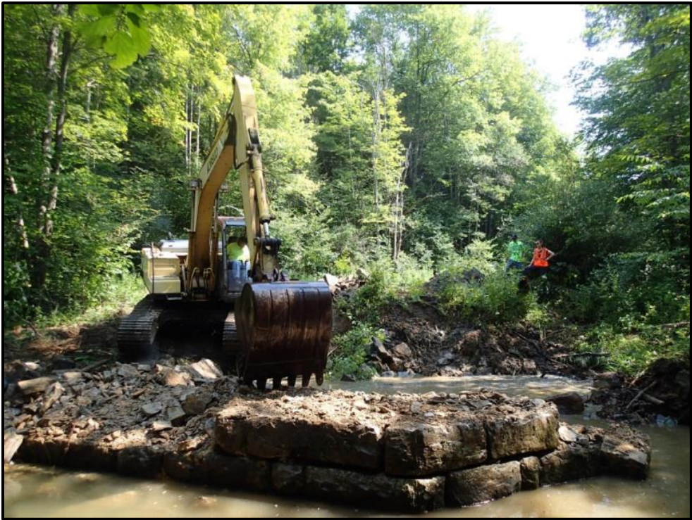
Figure 7 - Deconstructing the stone abutment.
