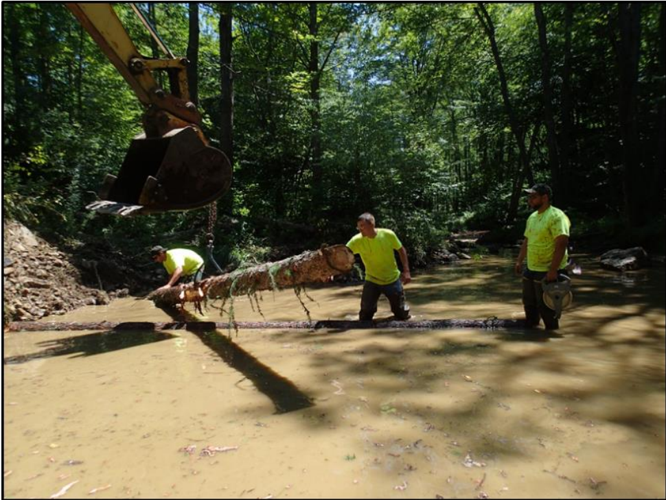
Figure 9 - Constructing the mud sill.
