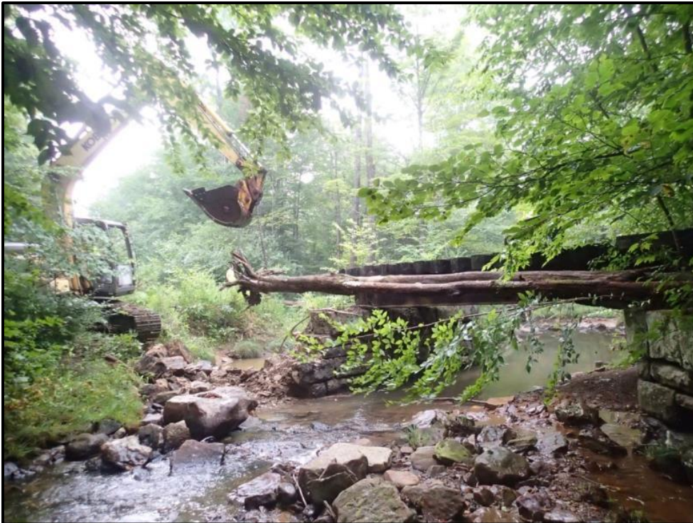
Figure 6 - Removing the old railroad bridge pier.
