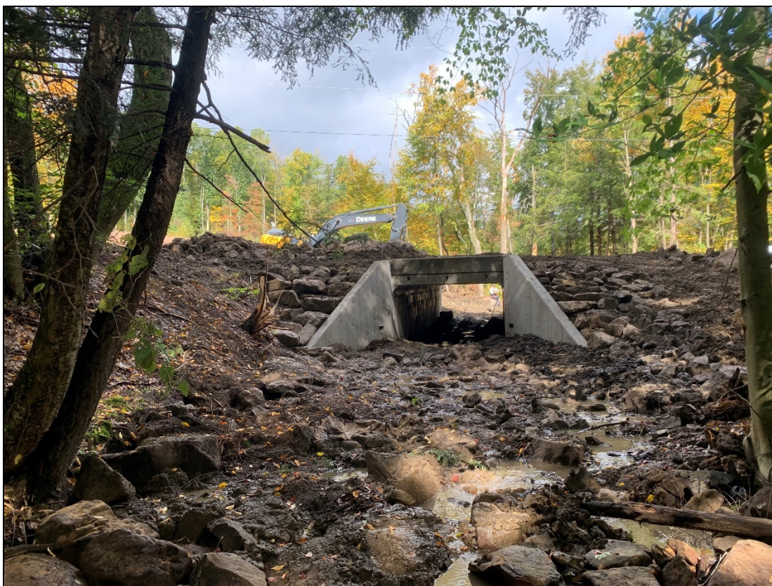
Figure 8 - Post installation view of Sidney Road box culvert
