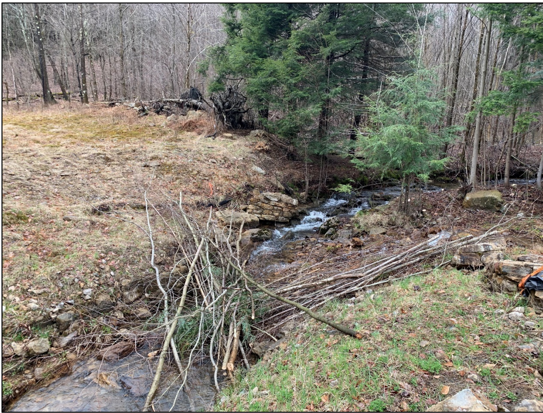
Figure 4 - Keal Run LWM brushing in progress
