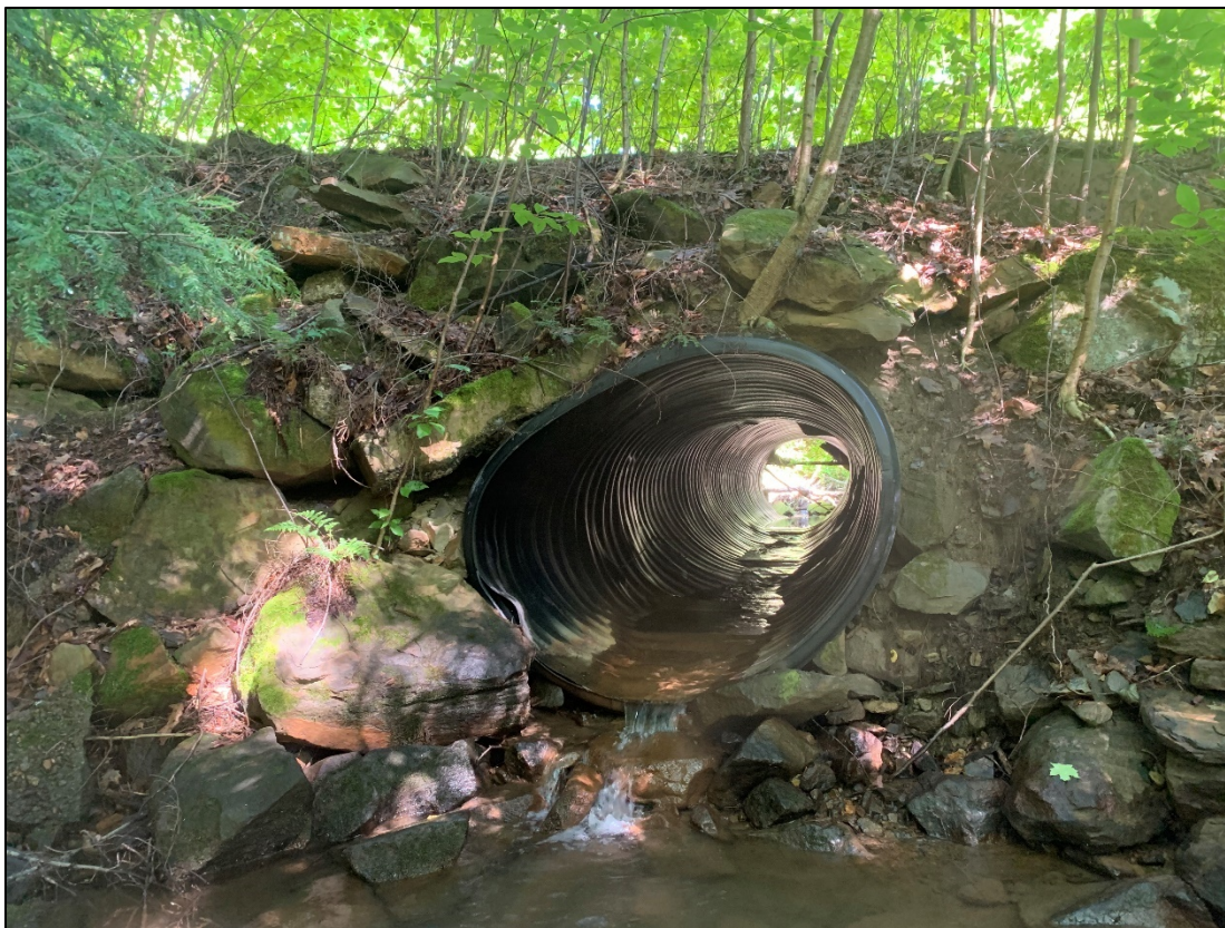
Figure 7 - Sidney Road culvert prior to AOP restoration
