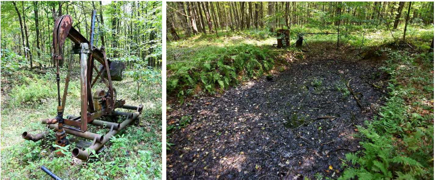
Figure 28. Inactive well site with pump jack (photo left) and old separator with overflow pit (photo right) in the Pithole Creek watershed.
