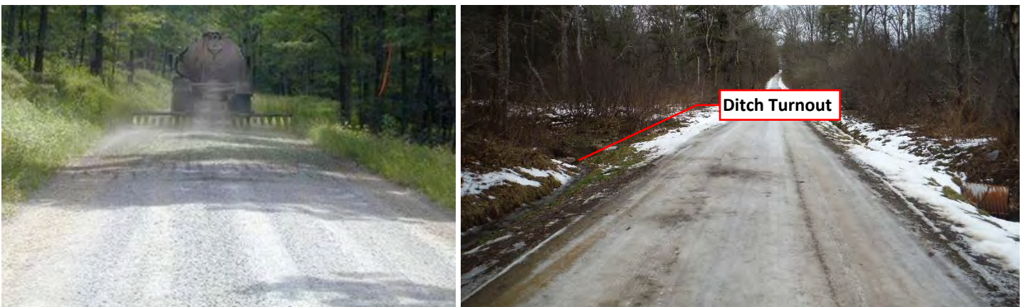
Figure 29. Typical application of brine on dirt and gravel roads as practiced prior to 2018 (photo left) and ditch turnout on Dean Road aiding brine and sediment runoff into Otto Run (photo right).
