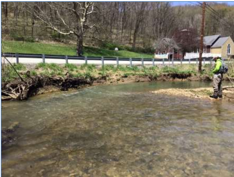
FIGURE 18 – ROAD ENCROACHMENT AND EROSION NEAR BENS CREEK LUTHERAN CHURCH
