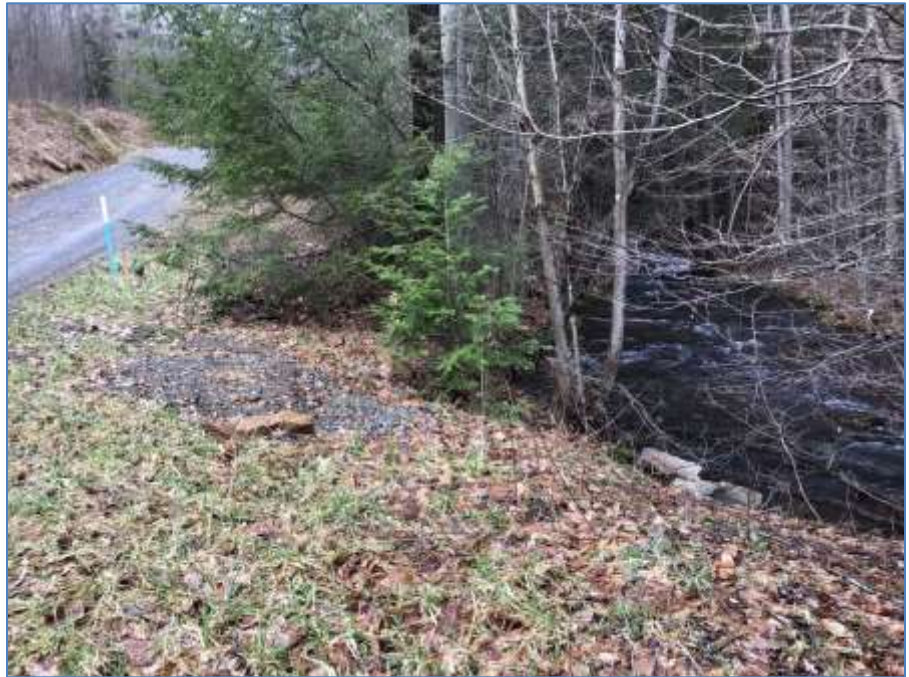
FIGURE 11 - DGR ACCESS ROAD ENCROACHING ON SOUTH FORK HEADWATERS
