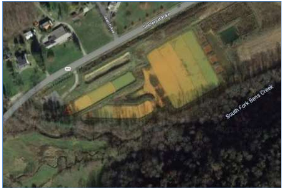
FIGURE 13 - LION MINE PASSIVE TREATMENT SYSTEM (PHOTO: GOOGLE)
