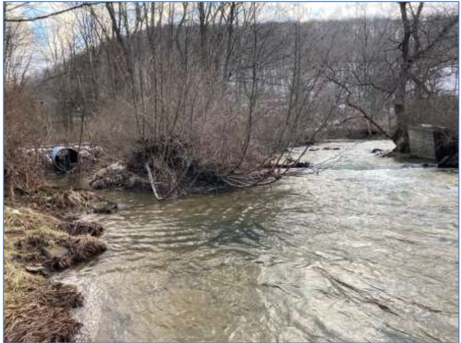
FIGURE 19 – UNPERMITTED AND ABANDONED STREAM ENCROACHMENT ON SOUTH FORK
