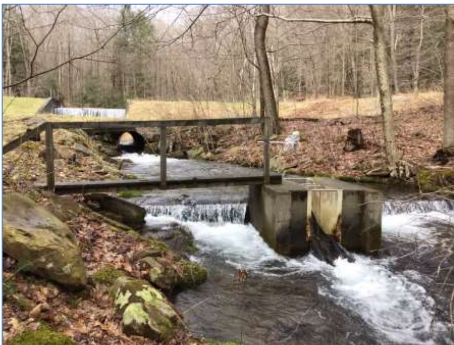
FIGURE 10 - MULTIPLE AOP BARRIERS AT OLD DAM SITE
