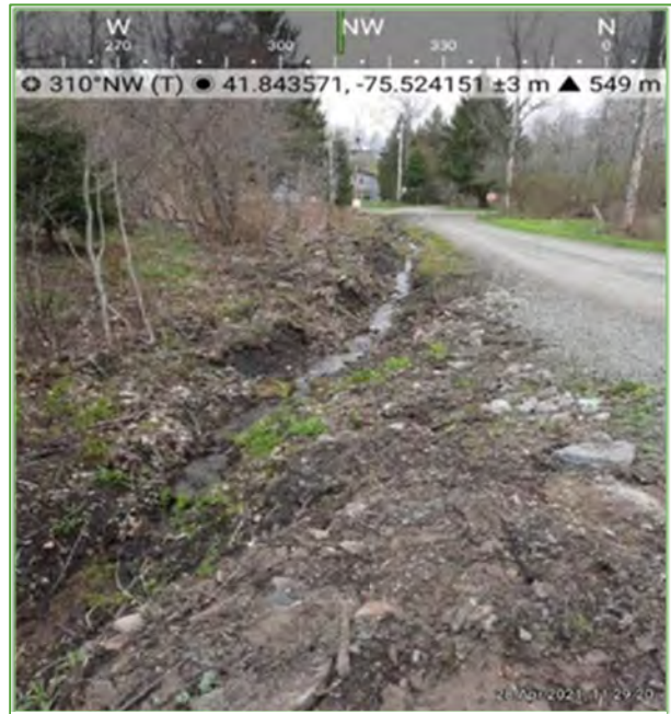
Figure 30 Ogden Road Ditch
