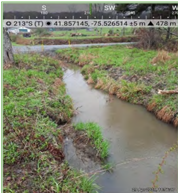
Figure 29 Ararat Road ditch
