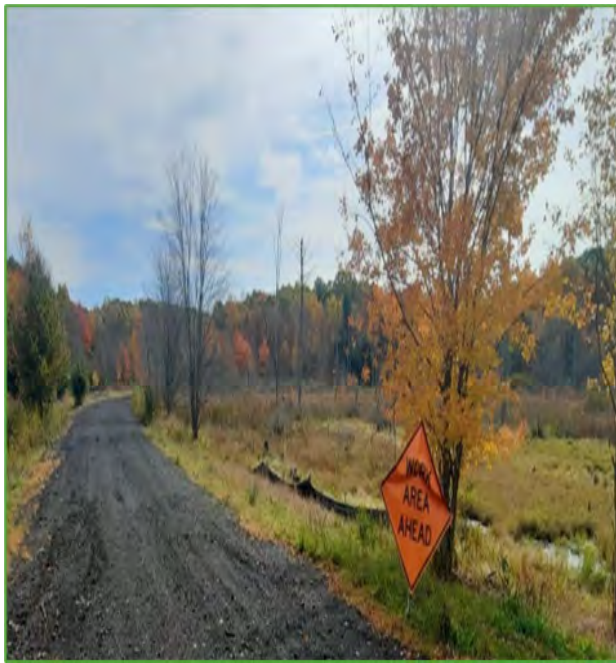
Figure 25 Rail Trail maintenance resulting in degraded habitat scores
