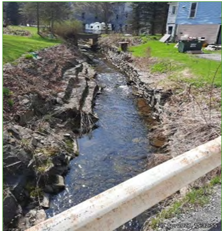
Figure 8 Starrucca Creek main stem below the Spencer mill dam in Thompson. Channel restriction due to armored banks.
