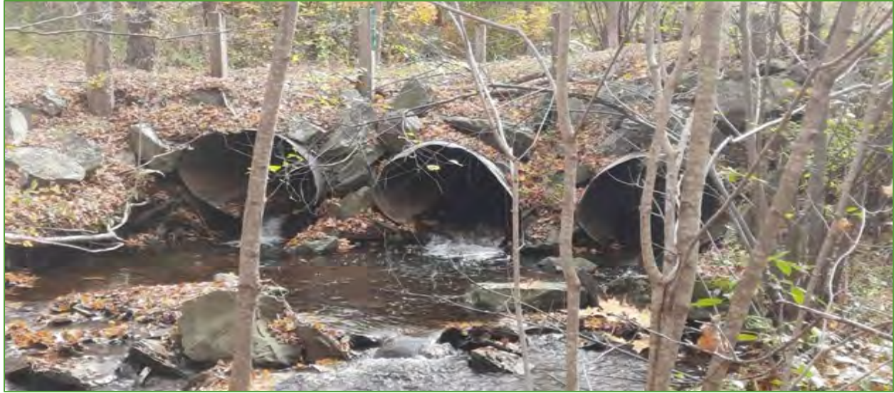
Figure 17 Crossing 92244 consisting of three elliptical pipes
